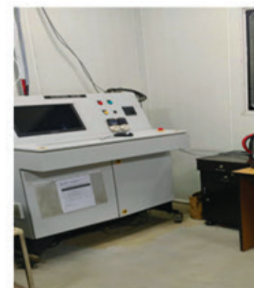
Master Controller for Combined System Test
