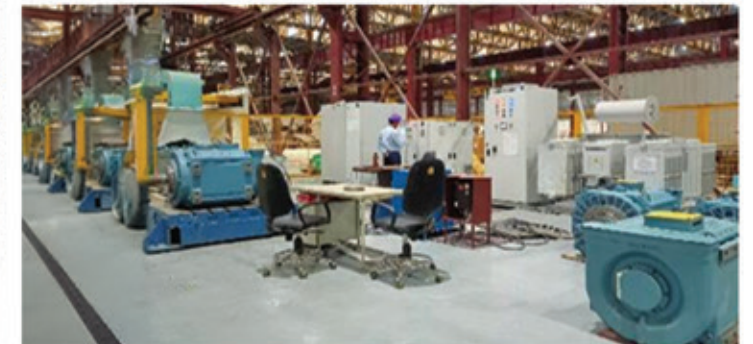
Traction Motor Testing Facility
