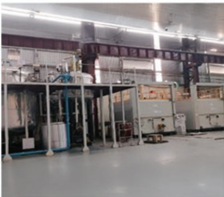
VPI Plant with Oven
