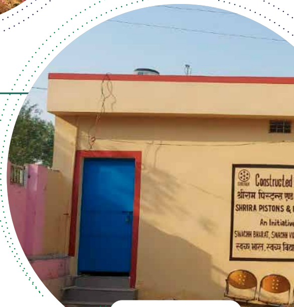
Toilet Built in School
