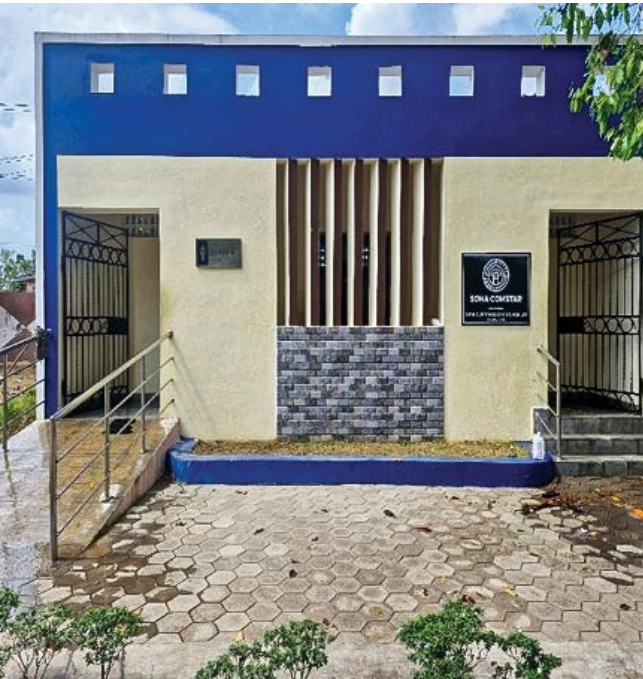
Figure 10: Toilets for Gents
