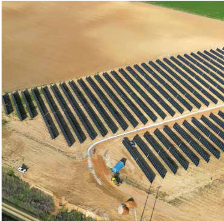
Solar farm in Medina, Spain.
