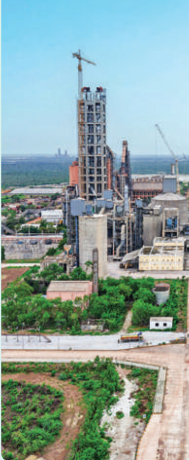
6-stage In-Line Calciner (ILC) preheater at Dacheipalli, A.P
