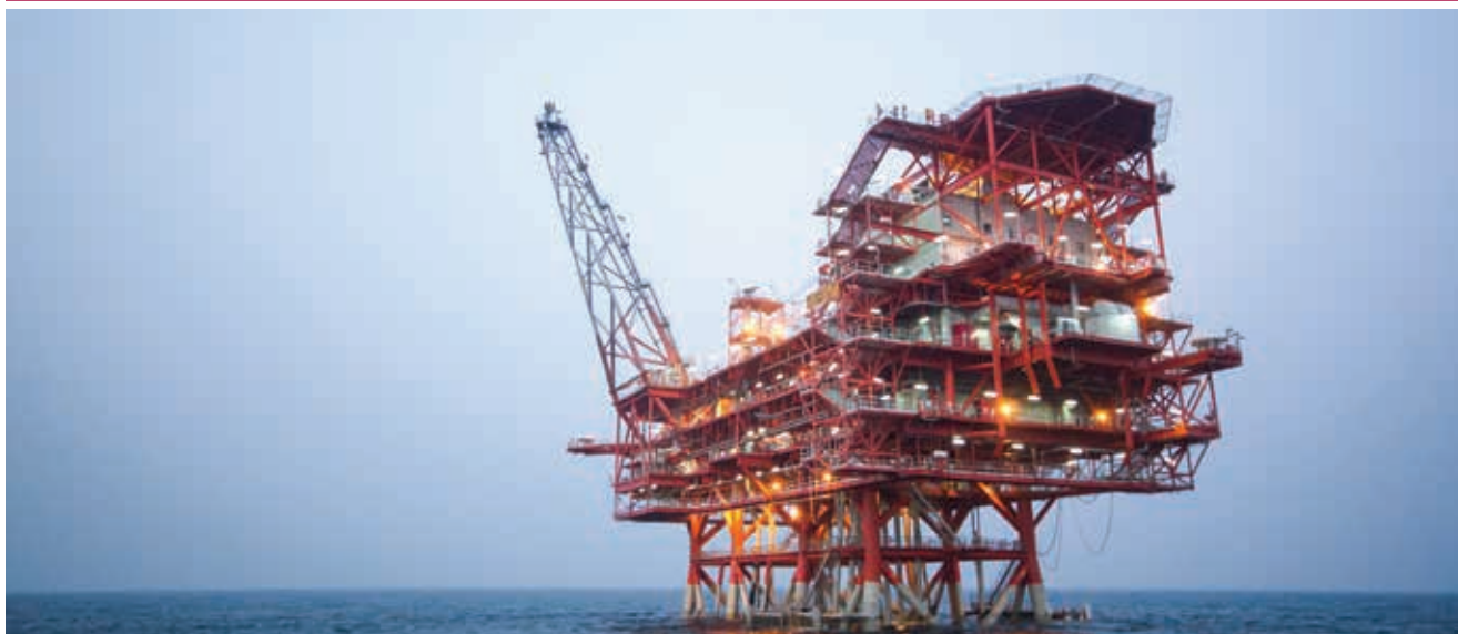
Control riser platform KG D6
