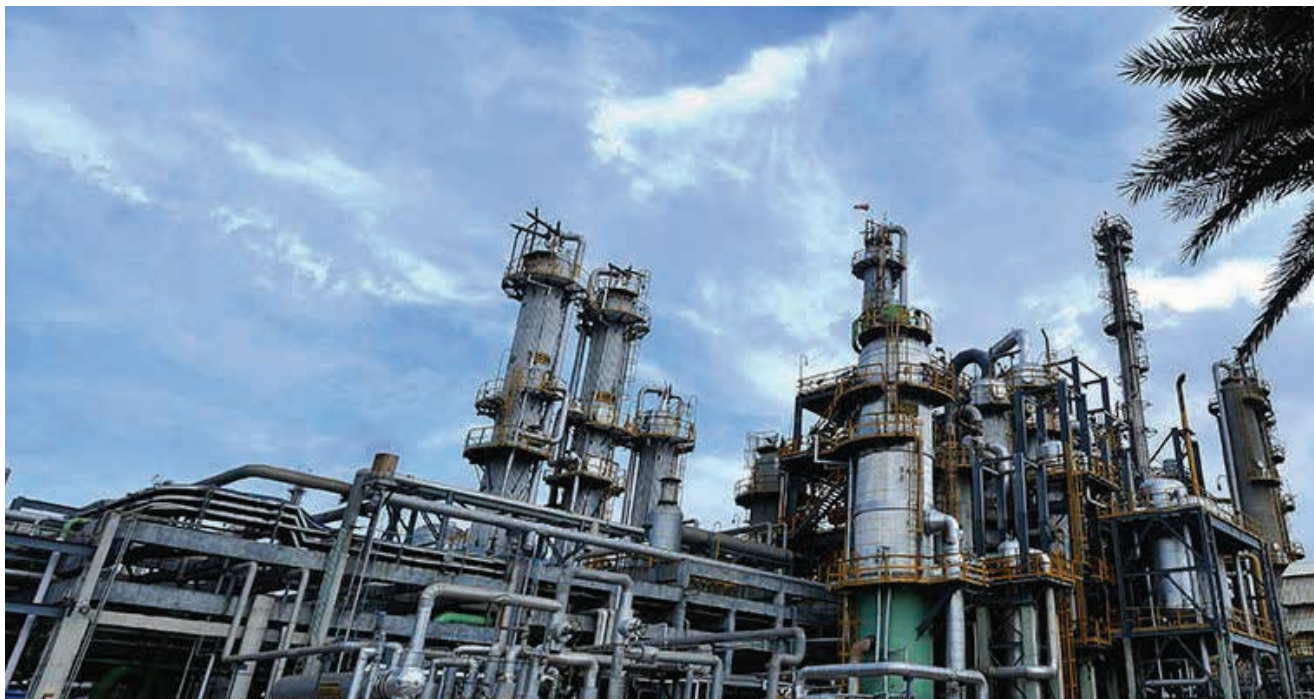
Petrochemicals Manufacturing Site
