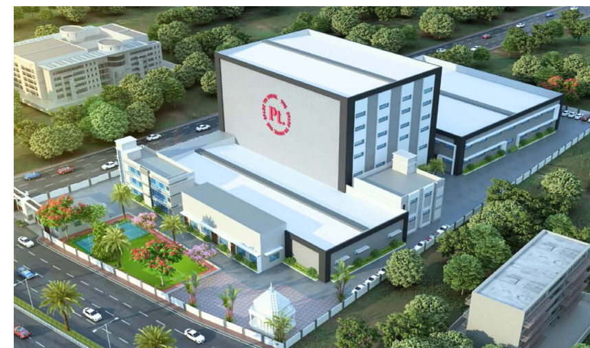
Palghar's expanded facility: nearing completion, enhancing sustainable capacity for global markets.
