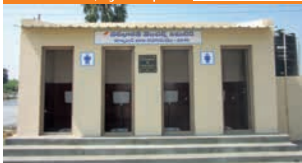
Toilet at ZPS School, Jagannadhapuram
