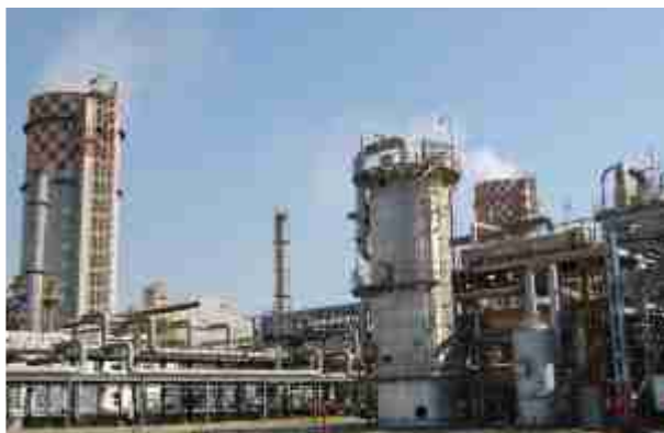
VIJAIPUR I & II PLANT
