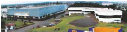
Menon Bearings plant at Kolhapur,
