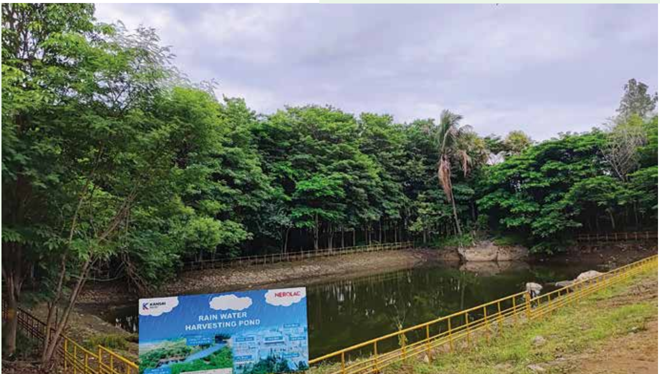
Rainwater Storage Tank at Hosur Plant
