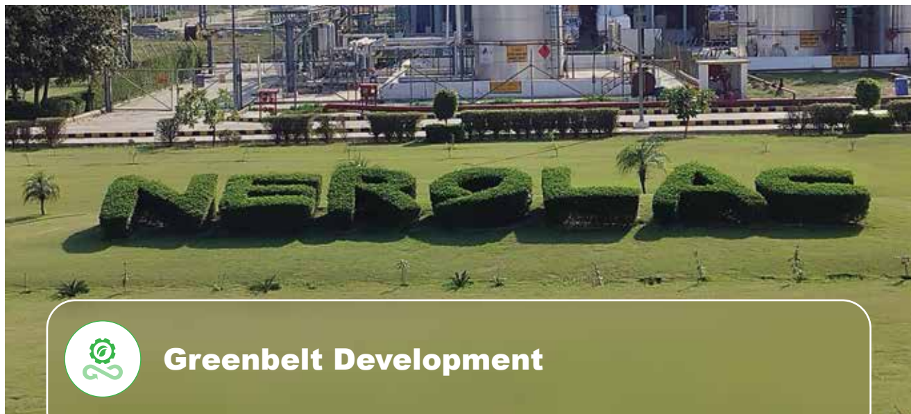
Greenbelt Development at the Goindwal Sahib Plant
