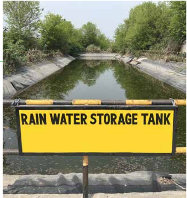
Rainwater Storage Tank at the Goindwal Sahib Plant
