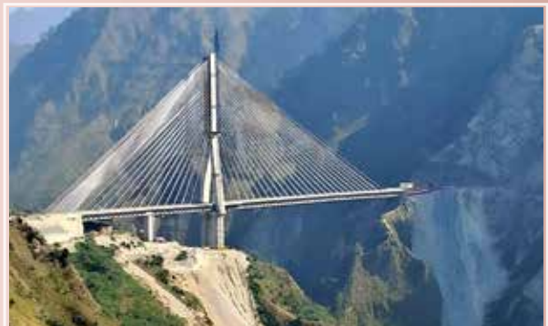
Anji Khad Bridge, Jammu & Kashmir
