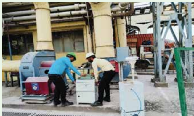
Installation of Air Handling Units at the Jainpur Plant
