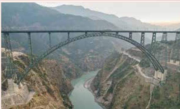
Chenab Bridge, Jammu & Kashmir (World's Highest Railway Bridge)
