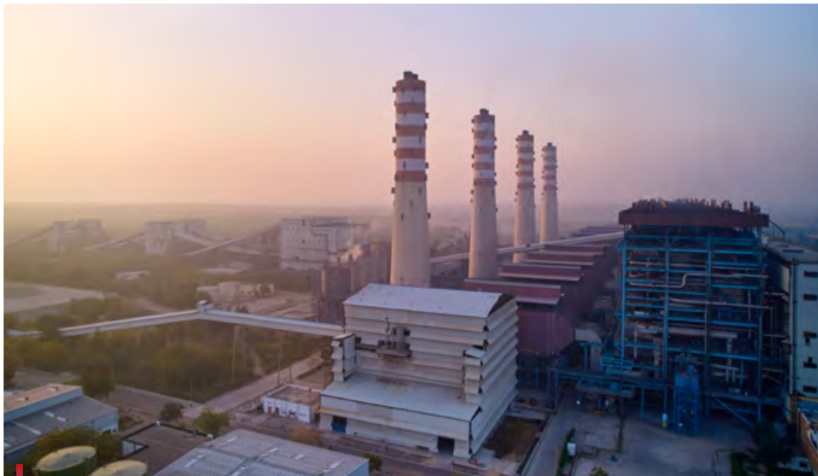
Thermal Power Plant, Barmer
