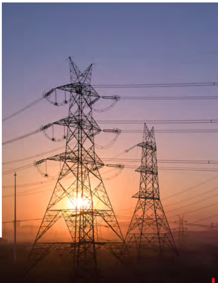
Power Transmission Line, Ratnagiri
