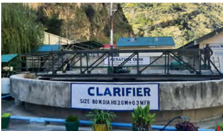
Water Treatment Plant, Sholtu
