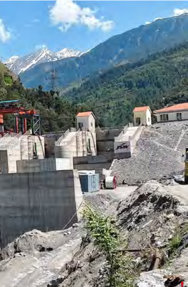
Kutehr Hydro Project
