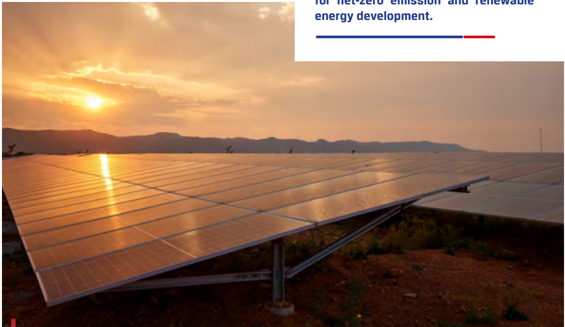
Solar Power Plant, Vijayanagar
