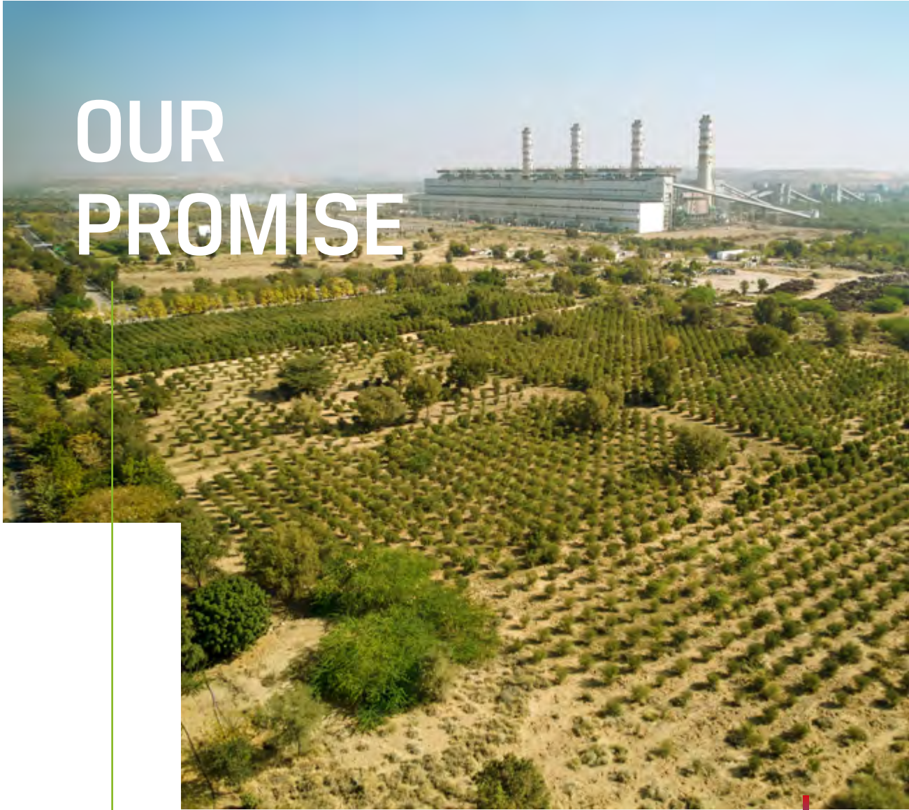
Barmer Thermal Plant
