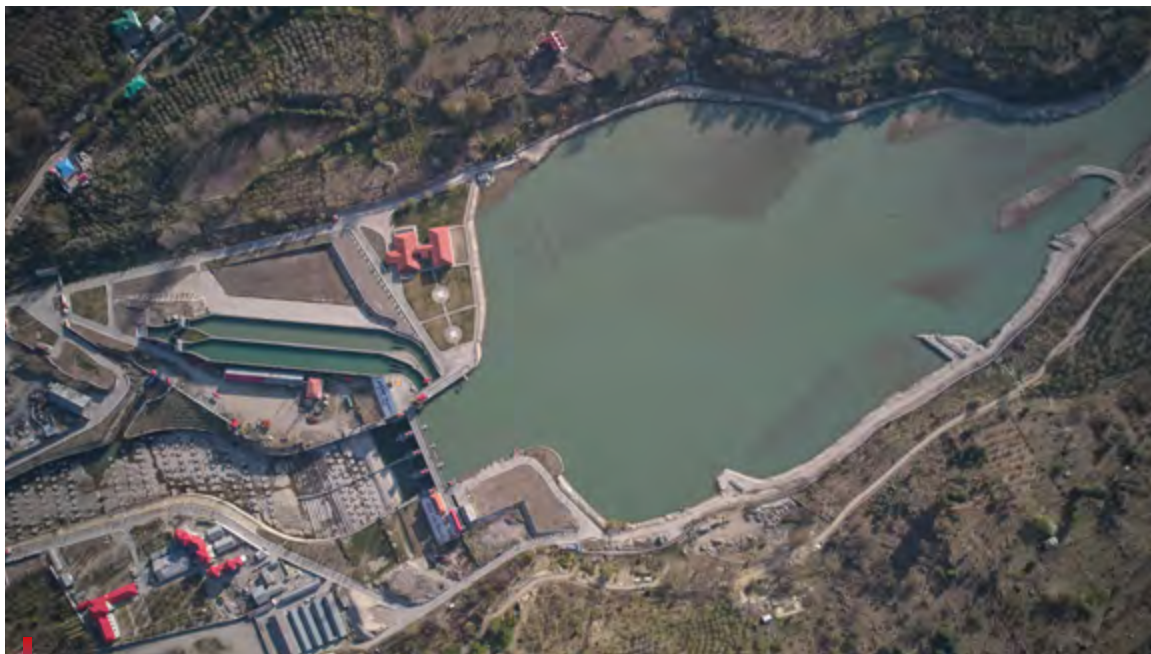
Hydro Power Plant, Sholtu
