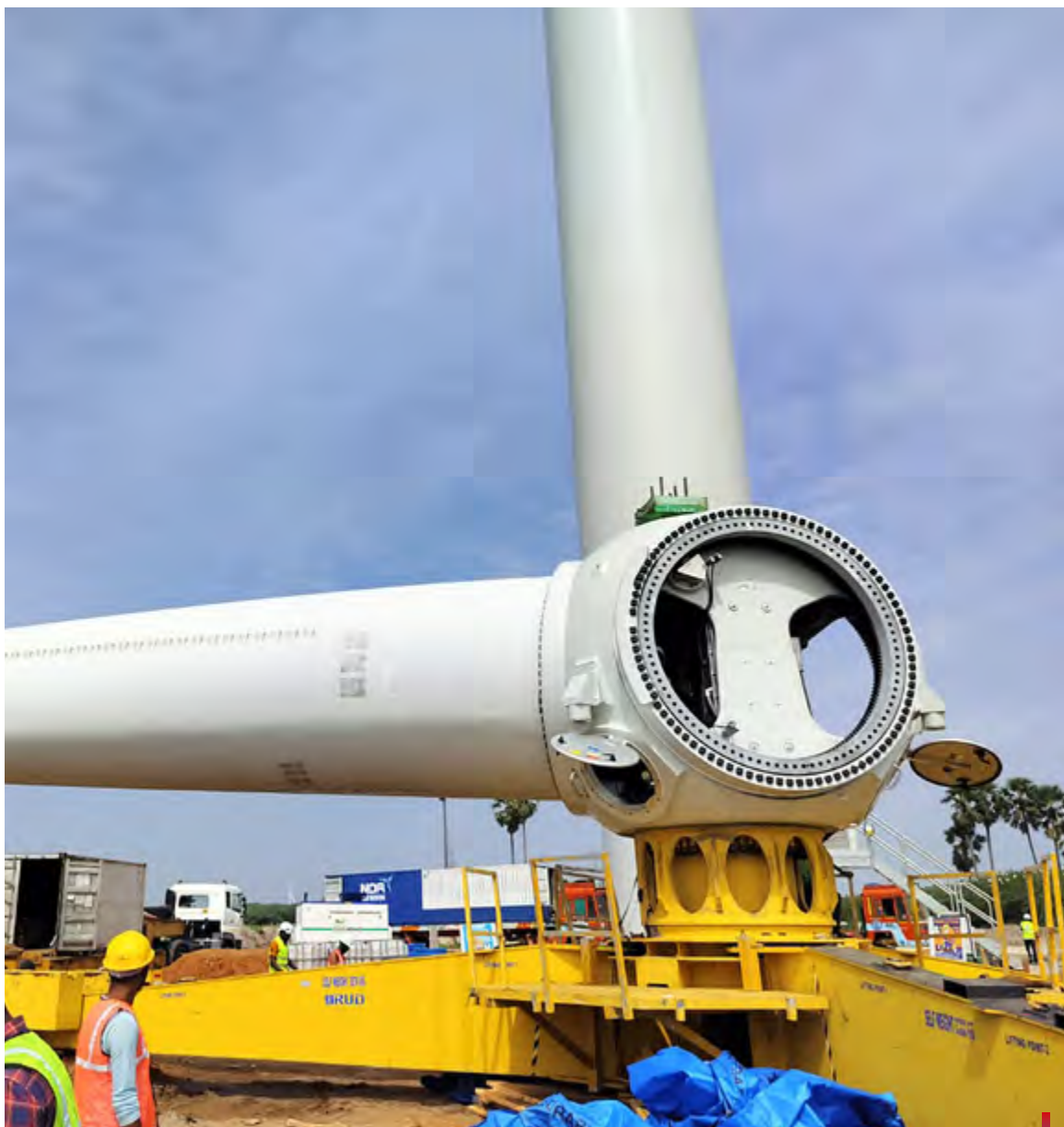
Wind Turbine Construction at Tuticorin Project
