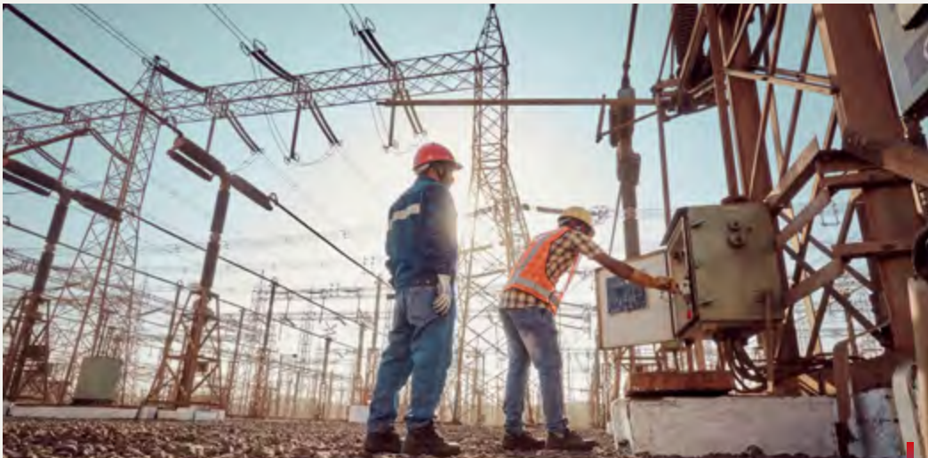
Switch yard, Vijayanagar Plant
