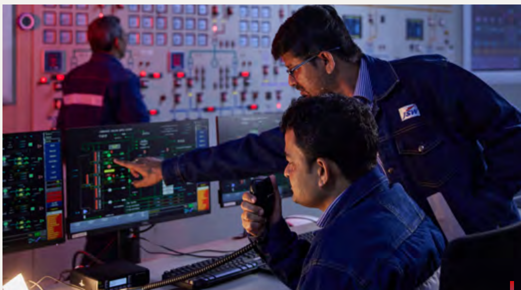
Thermal Power Plant, Vijayanagar
