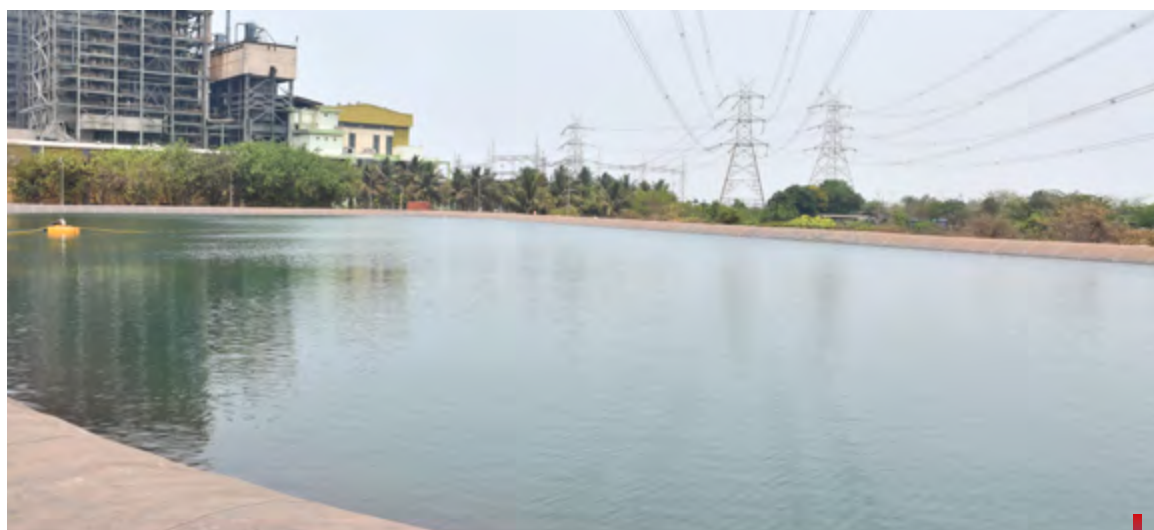
New Water Reservoir at Ratnagiri Plant
