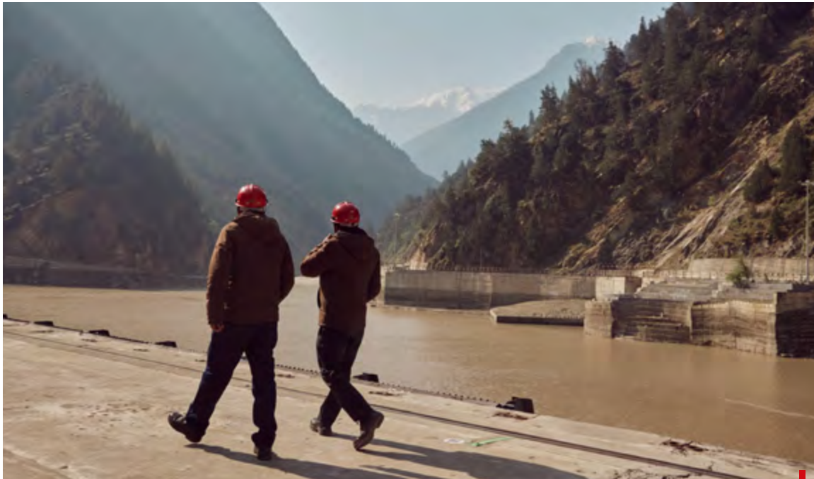
Karcham Dam, JSW Hydro Sholtu
