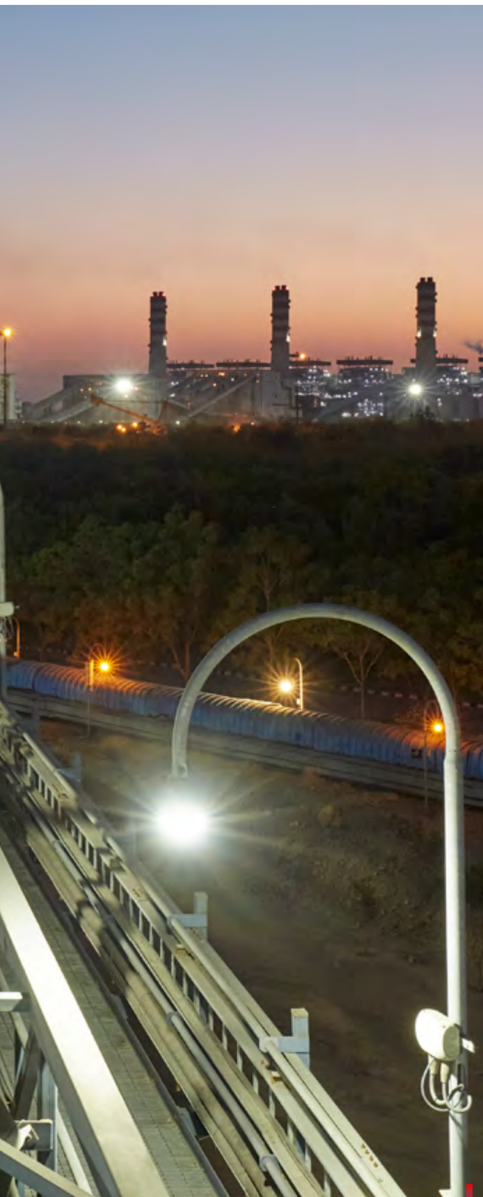
Barmer Power Plant
