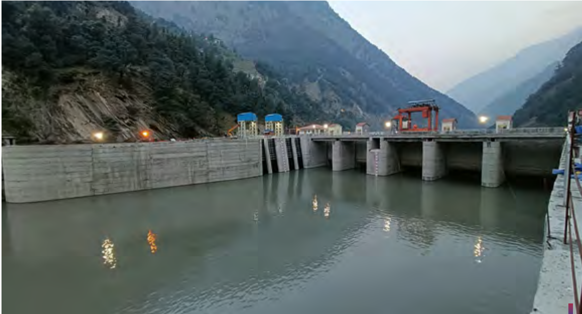
Barrage, Kutehr Hydro Project
