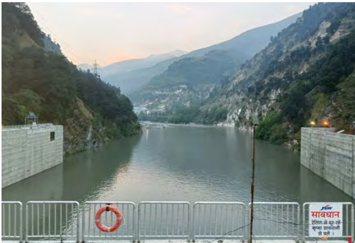
Kutehr Hydro Project
