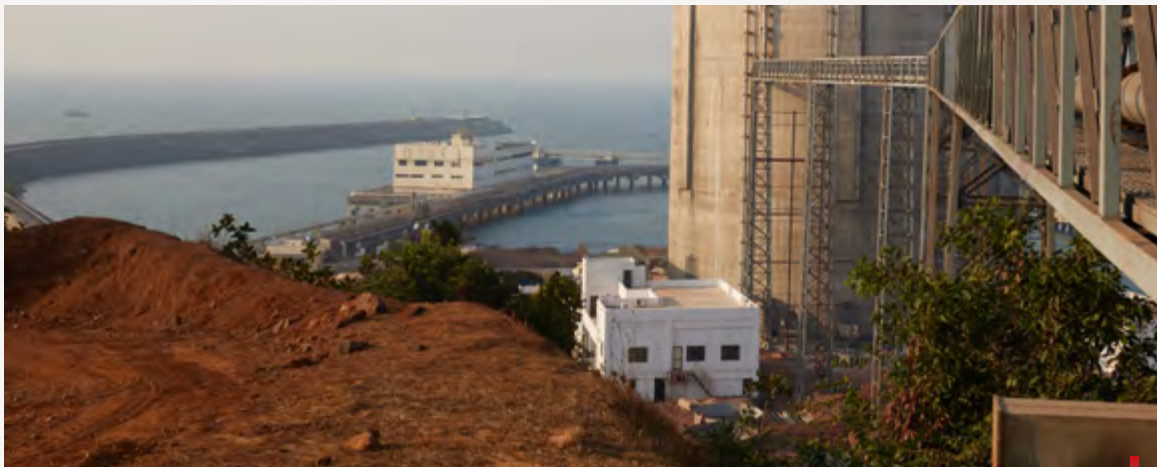
Fly Ash Silo at Ratnagiri Plant
