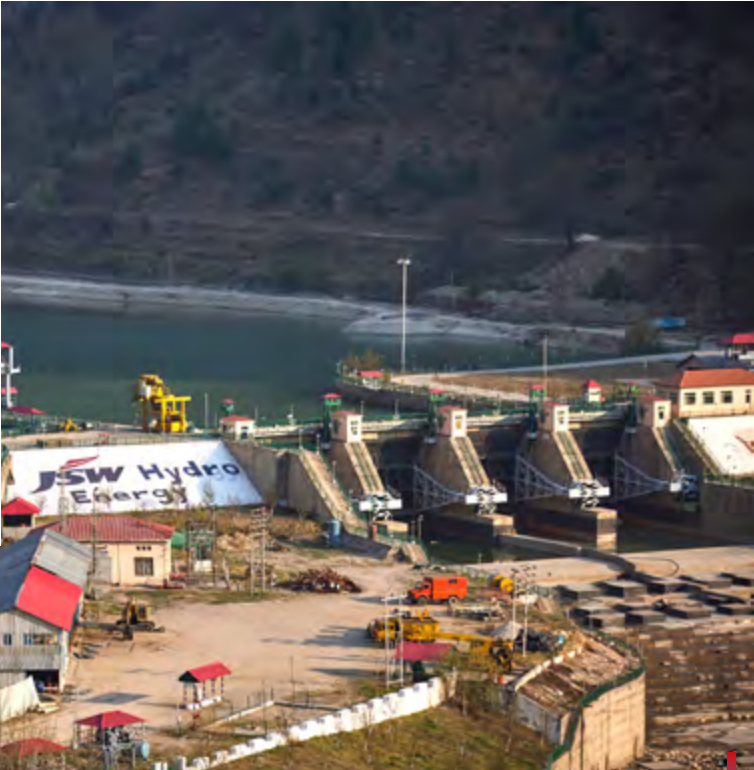
JSW Hydro Energy, Sholtu
