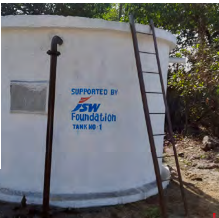
Nandiwade Kunbiwadi Water Tank for Ratnagiri Community
