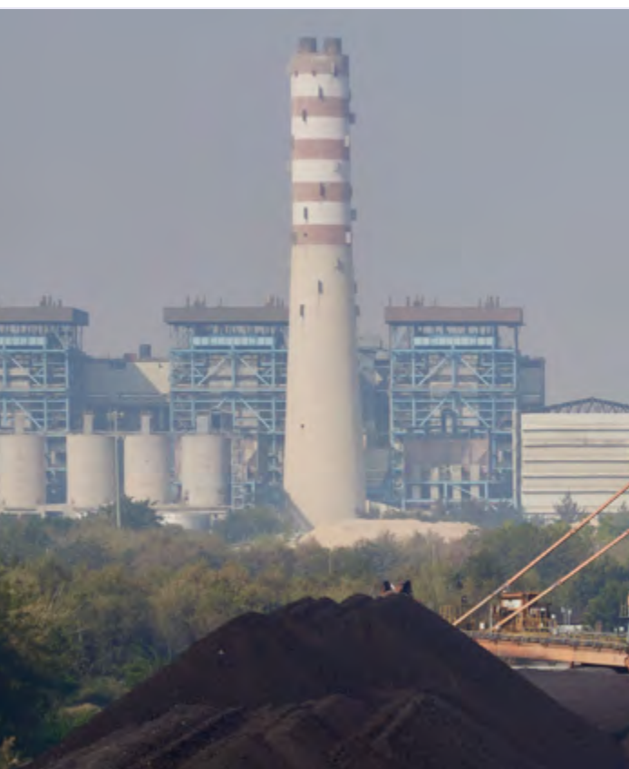
Power Plant, Utkal
