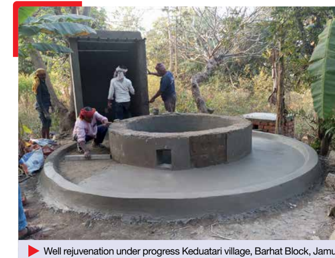
▶ Well rejuvenation under progress Keduatari village, Barhat Block, Jamui
