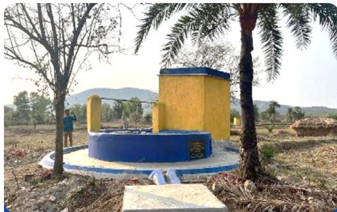
Rejuvenated well and bath shed ready for handover
