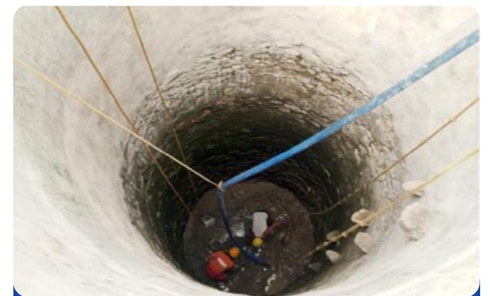
Well cleaning and desilting in progress
