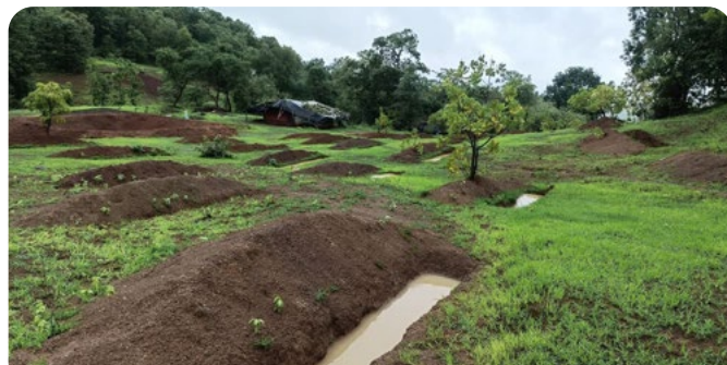
Continuous Contour Trenches dug along hill slopes
