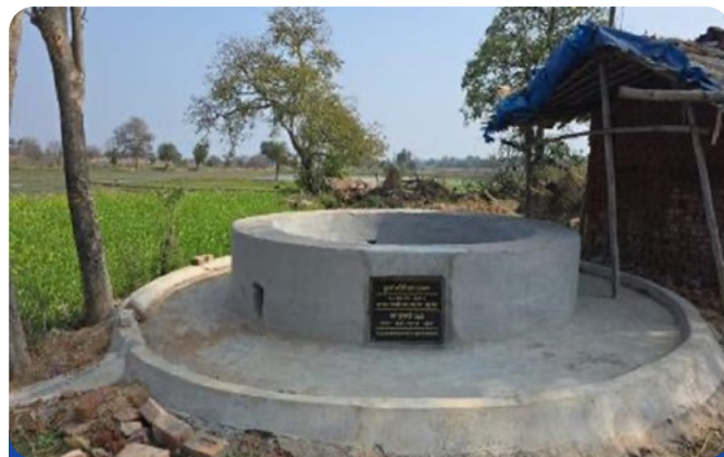
Well cementation and platform construction completed
