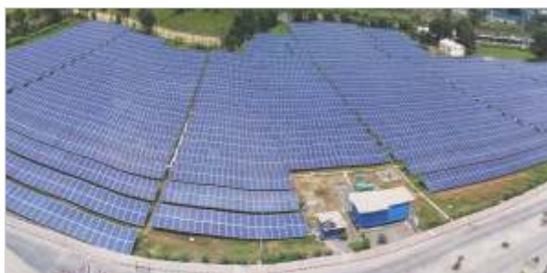
Surat Grinding Unit has commissioned 2.36 MW captive solar power plant that meets about 12 % of the total power requirement of the Unit
