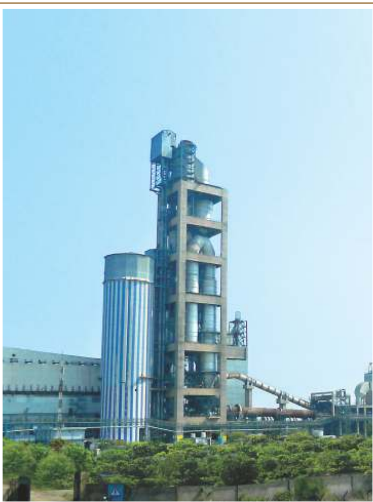
Integrated Cement Unit, Durg
