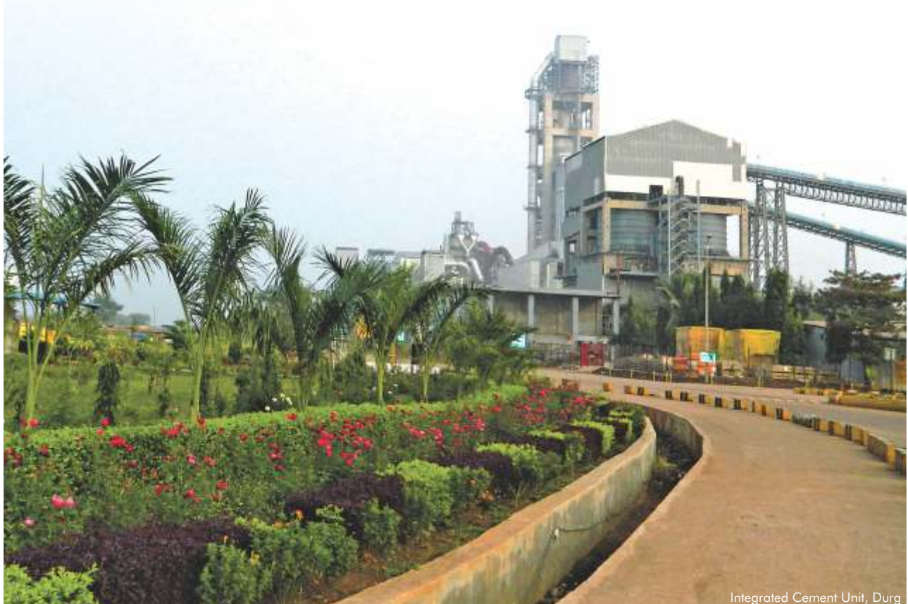
Integrated Cement Unit, Durg
