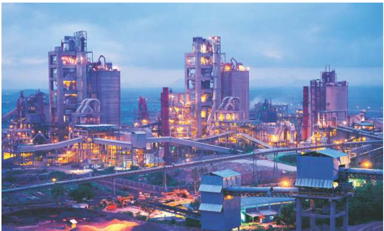
Integrated Cement Unit, Sirohi
