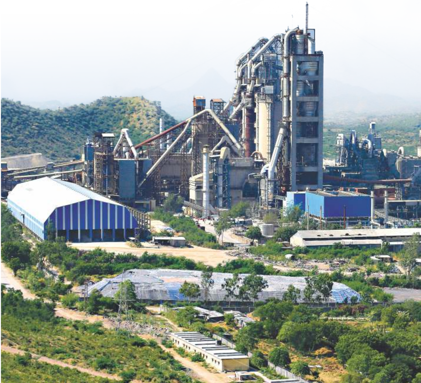
Integrated Cement Unit, Sirohi
