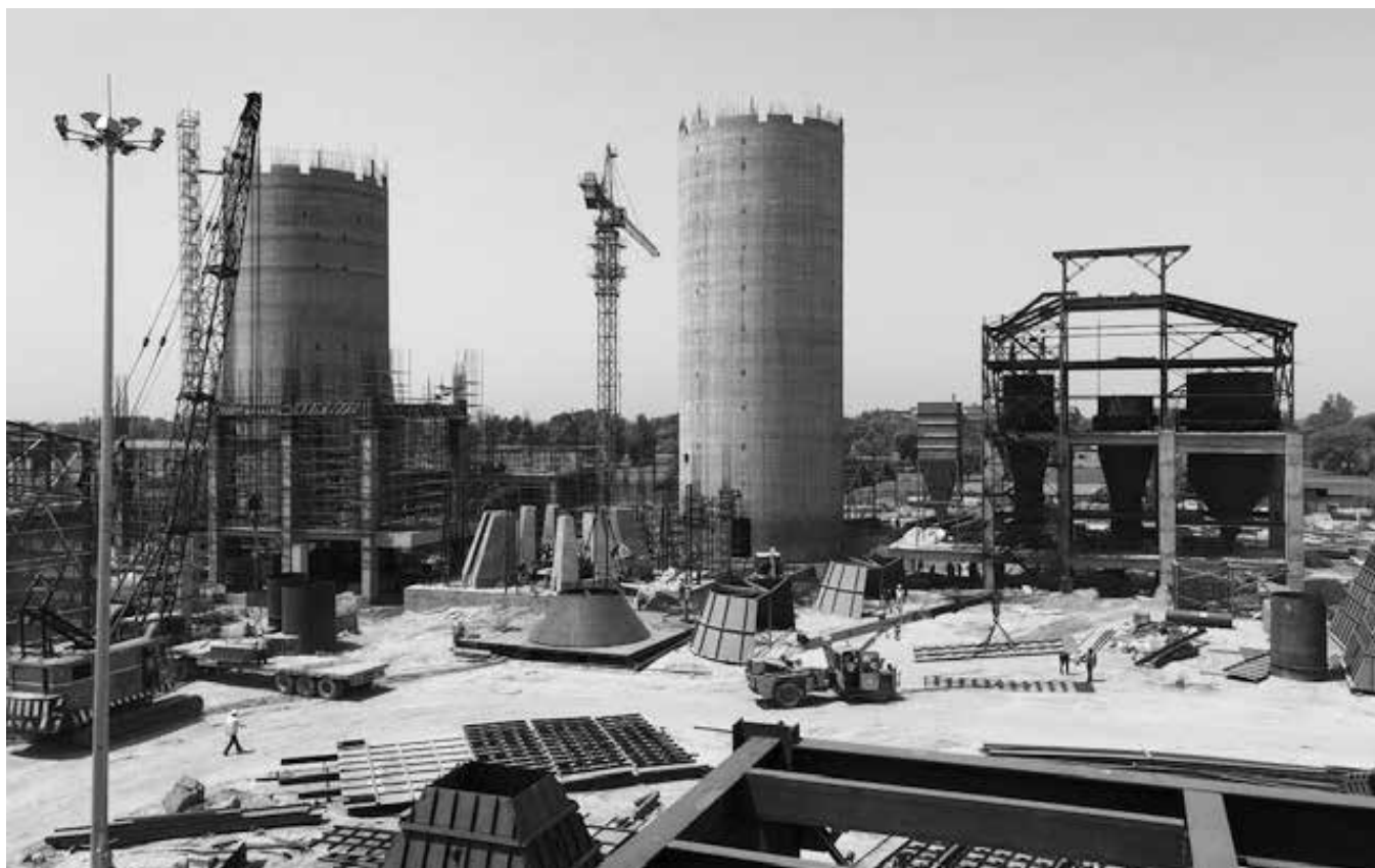
Aligarh Grinding Unit (Greenfield Expansion)
