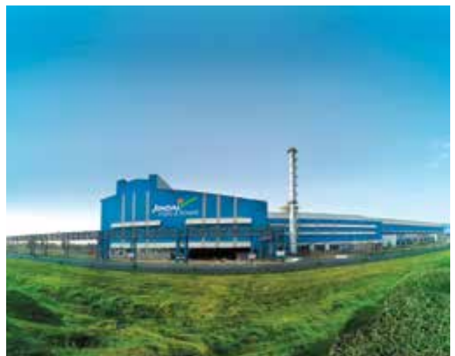
> 1 MTPA Rebar Mill at Patratu, Jharkhand
