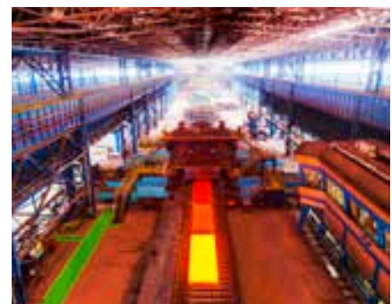
▶ 1.2 MTPA Plate Mill at Angul, Odisha
