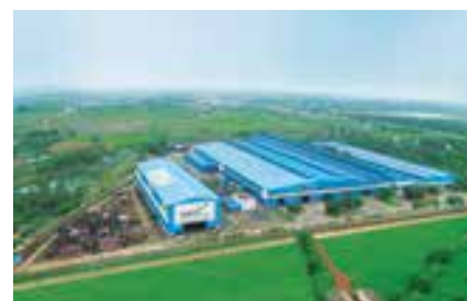
> Machinery Division at Raipur, Chhattisgarh
