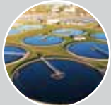
Water Treatment & Desalination
