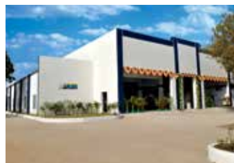
Drip & Sprinkler Irrigation Systems and Plastic Piping: Jain Plastic Park, Bhavnagar, Gujarat (India)
