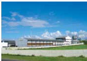
Drip and Sprinkler Irrigation Systems, Plastic Piping: Jain Plastic Park, Kondamadgu, Andhra Pradesh (India)
