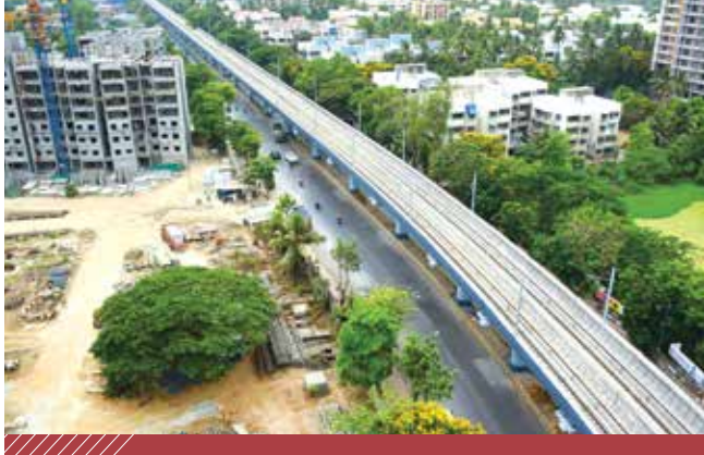
Mumbai Metro Line 2
