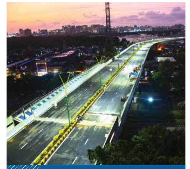
BKC- Chunabhatti Flyover
