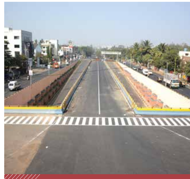
KSB Underpass, Pune
