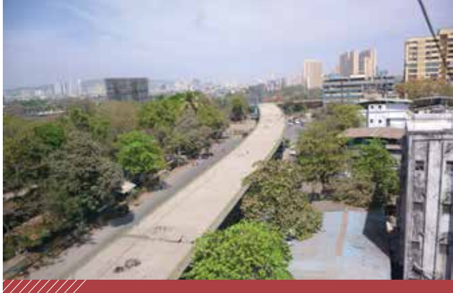
Kalwa Bridge Thane
