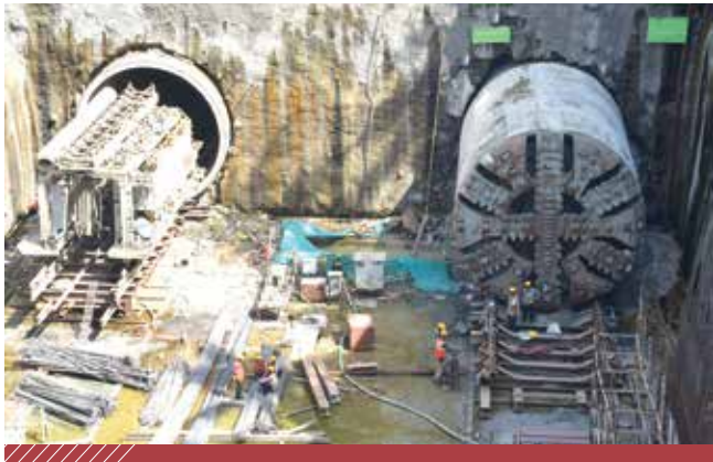
Mumbai Metro Line 3 Package 5 Vidyanagri South Retrieval Shaft
