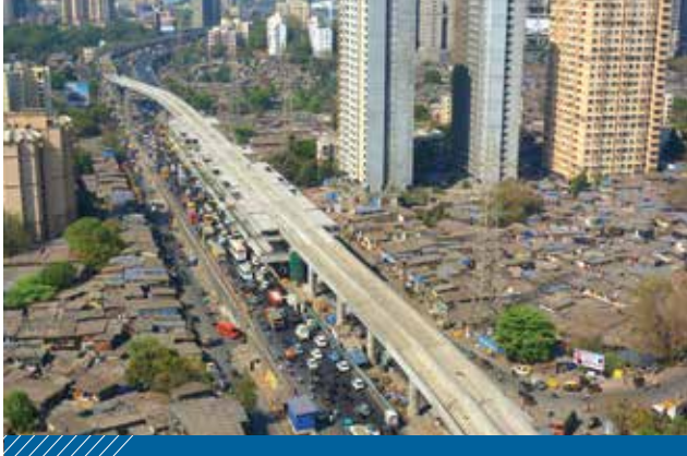
Mumbai Metro Line 7
