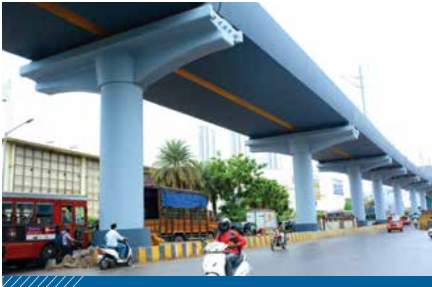
Mumbai Metro Line 2
