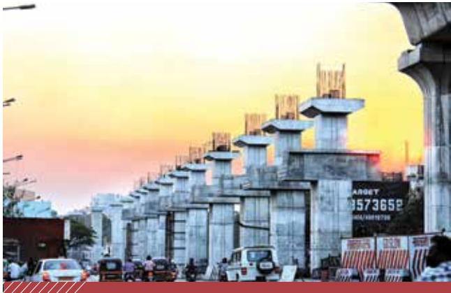
Pune Elevated Metro
