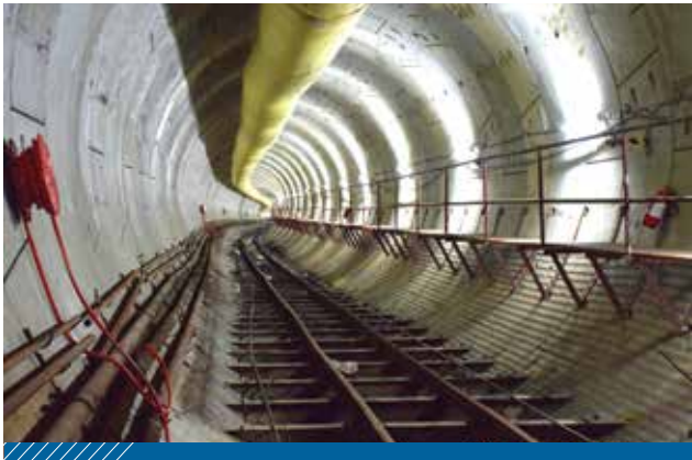
Mumbai Metro Line 3 Package 5 (BKC-Vidyanagri - Up line)
