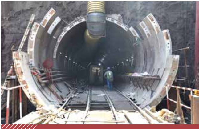
Mumbai Metro Line 3 Package 6
