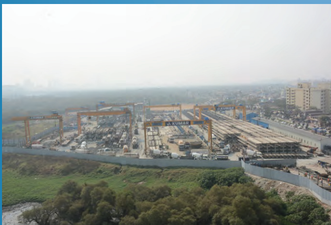
Malwani Casting Yard
