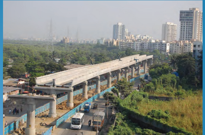
Mumbai Metro Line 2
