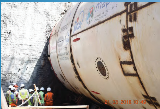
Mumbai Metro Line 3 Initial Drive
