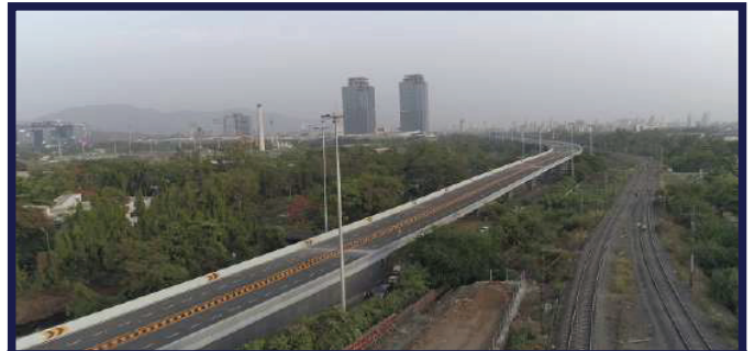
Thane Belapur Flyover
