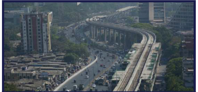
Mumbai Metro - Line 7
