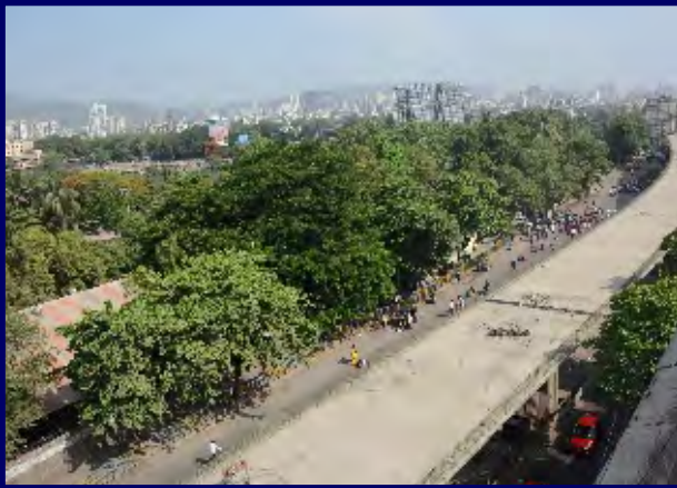
Kalwa Creek Bridge
