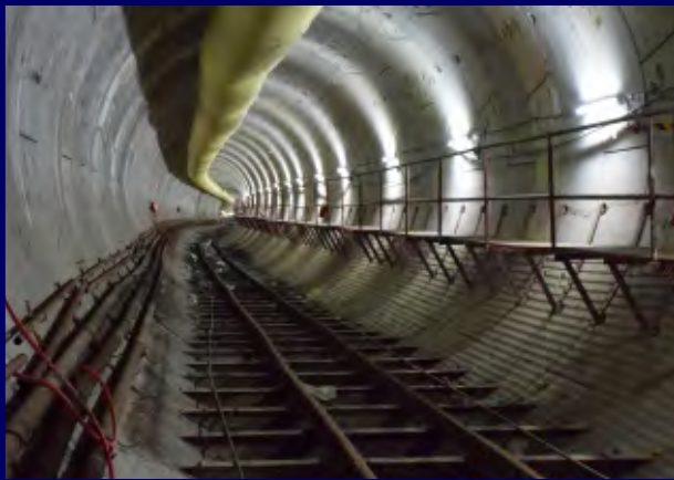
Tunnel From BKC to Vidyanagri
