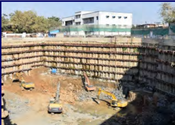
Sahar Metro Station at Mumbai
