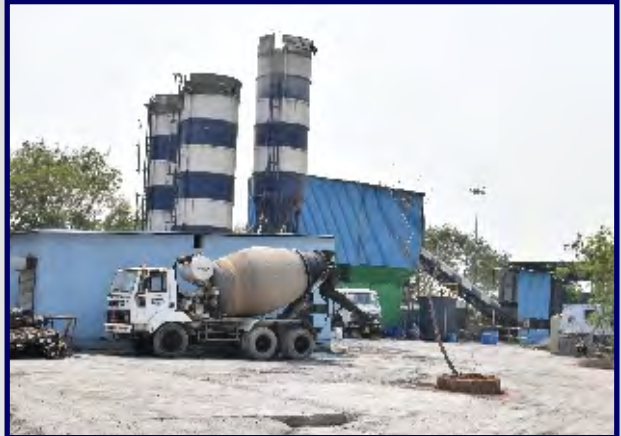
Ready Mix Concrete Plant
