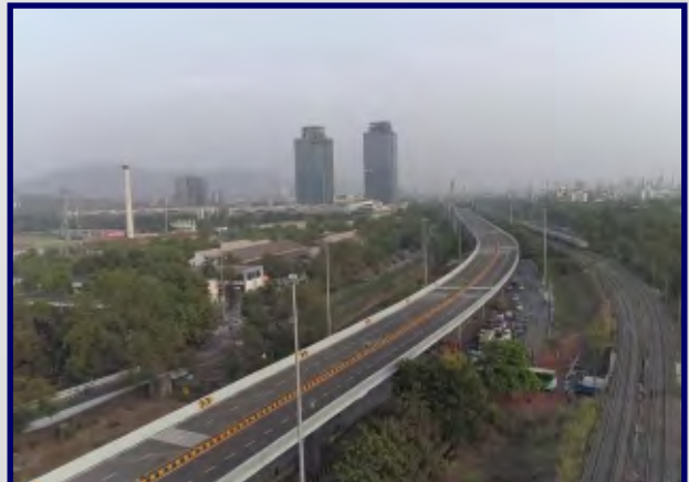
Ghansoli Flyover Navi Mumbai
