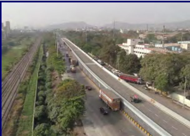
Thane Belapur Flyover
