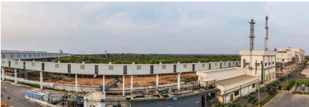
ITC's Integrated Consumer Goods Manufacturing Facility, Malur
