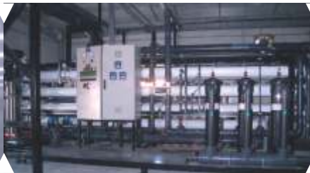
Reverse Osmosis Plant for Um Al Quain, UAE
