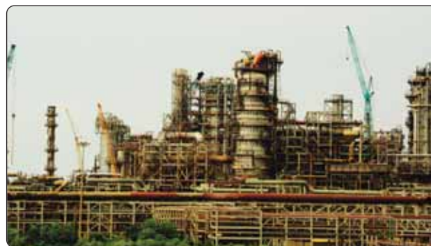
IndianOil's Paradip Refinery in Odisha under commissioning.
