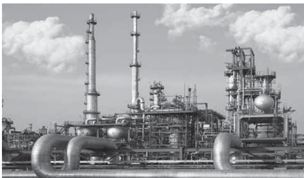
PX unit at Panipat Refinery
