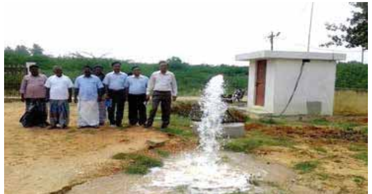
DRINKING WATER FACILITY AT DALAVOI
