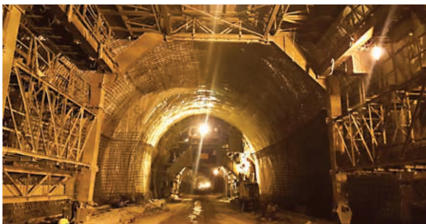
➤ Chenani Nashri Tunnel Project
