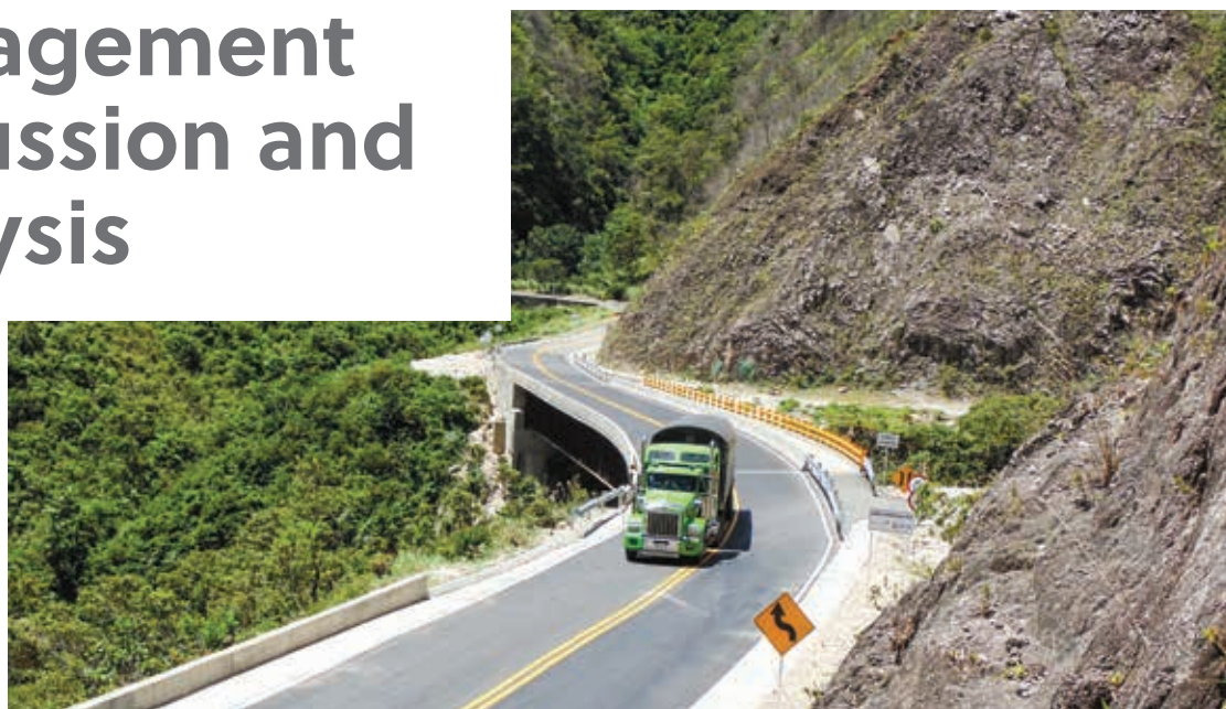
Colombia Bridge Project
