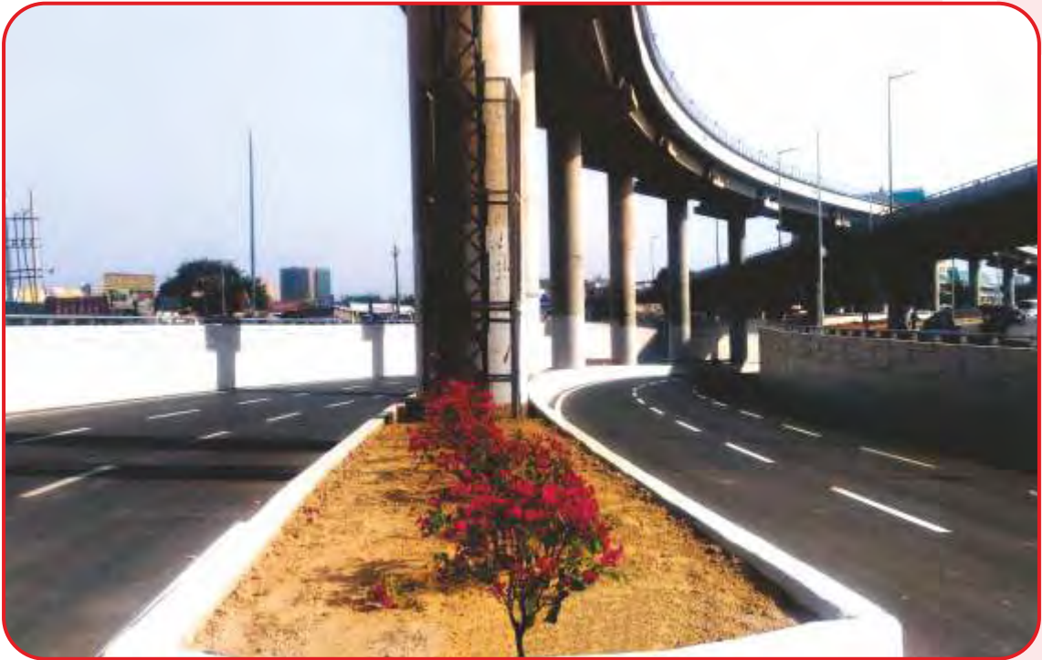
DLF Road Project, Gurgaon, Haryana
