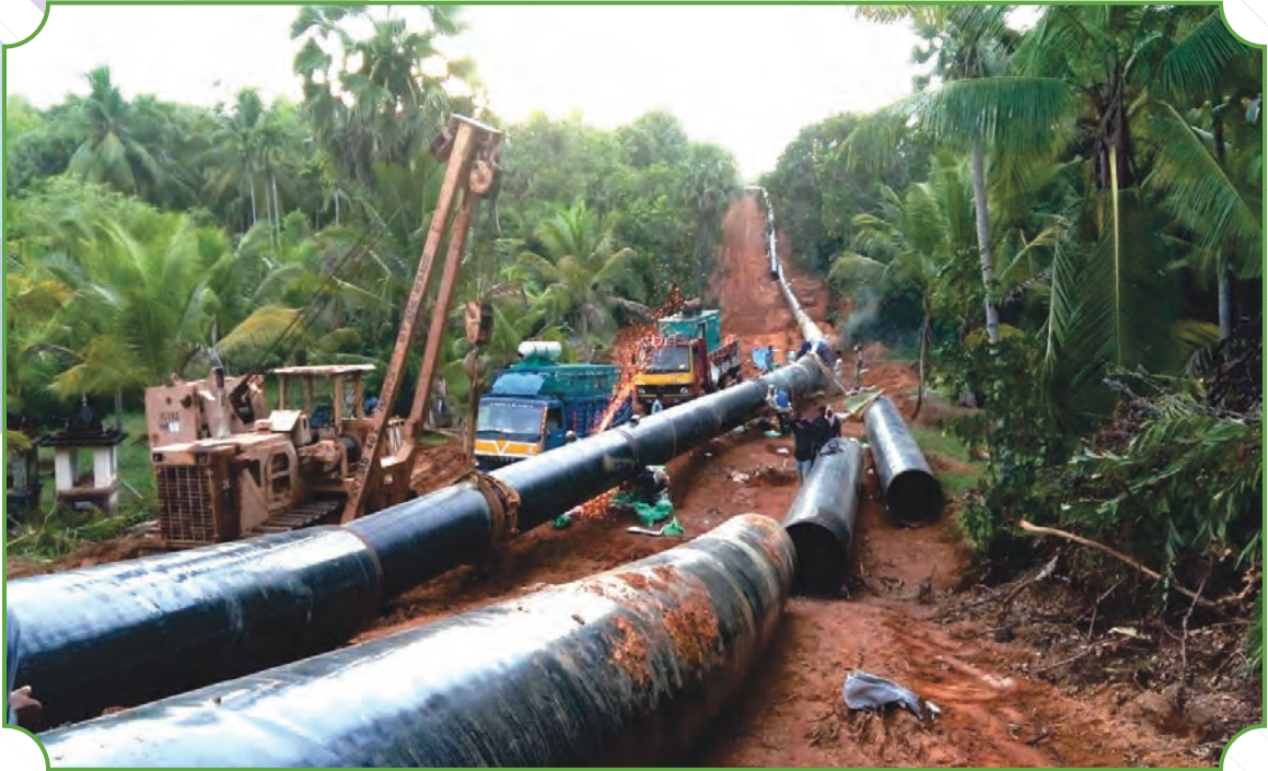
Mainline welding works for 42 inch pipeline as part of the EPC pipeline laying project for Indian Strategic Petroleum Reserves Ltd, Ministry of Petroleum & Natural Gas, Government of India in Mangalore, Karnataka
