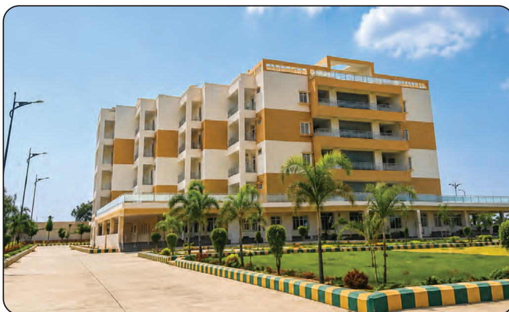
Integrated Township in Yadadri Thermal Power Station, Nalgonda, Telangana
