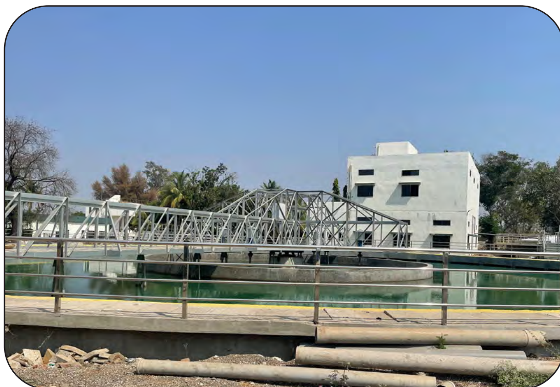
Clariflocculator through MUIF at Sambhaji Nagar, Mumbai
