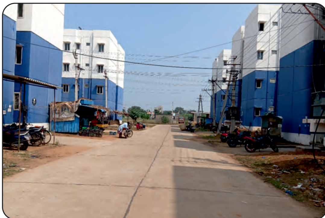
Construction of Housing Units under AHP Vertical of PMAY(U)-1.0, across Andhra Pradesh
