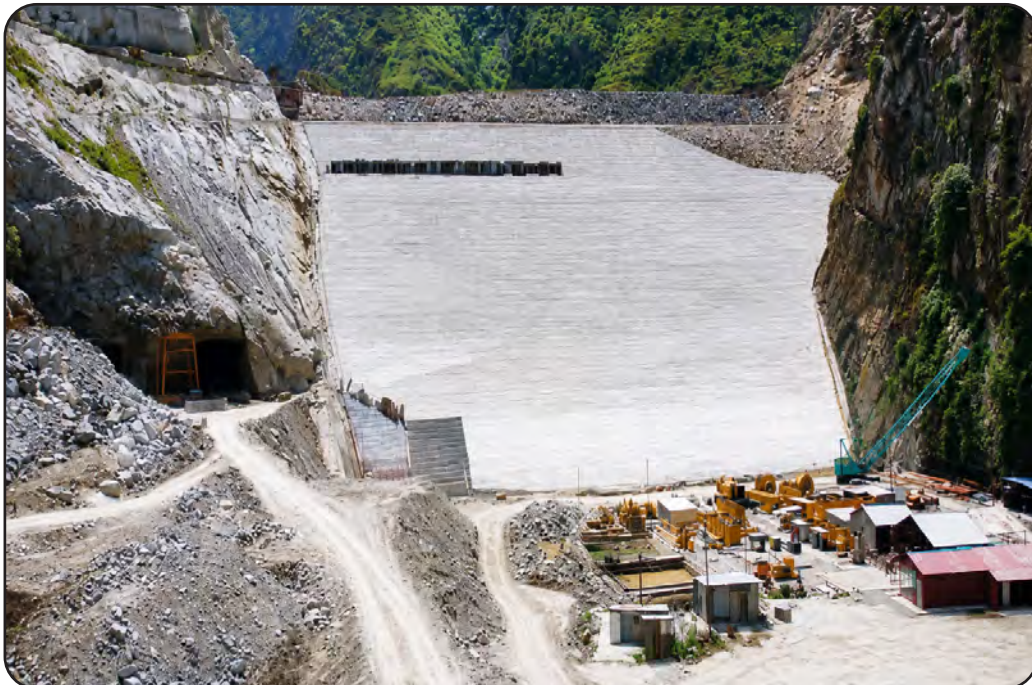
1000MW Hydroelectric Power Project at Pakal-Dul, Kishtwar, Jammu & Kashmir
