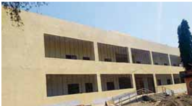
Construction of School Building, Nasik
