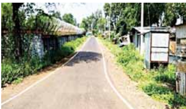
Service Road Repair, Nasik
