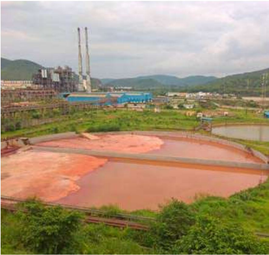
A caustic pond at Utkal Alumina. This pond re-circulates used caustic liquor from the Bayer process
