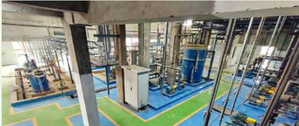
TWRU Pump house
