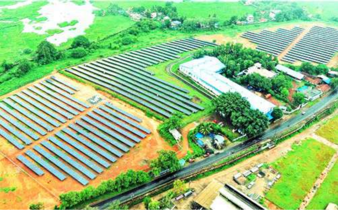
Solar Plant at Alupuram
