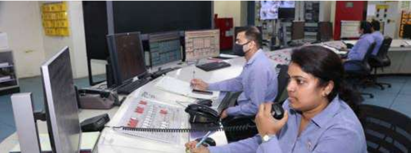
Power plant control room
