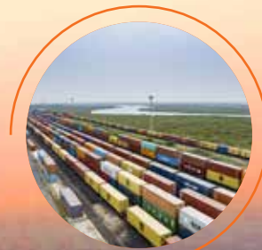
Dedicated Freight Corridor
