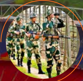
BSF's Modular Multi- Layered High-Strength Border Fencing
