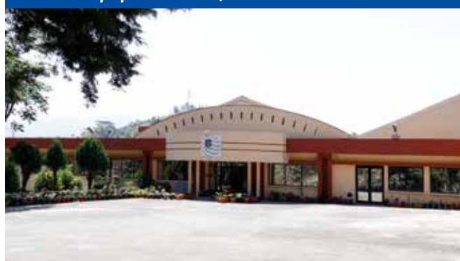
Telecom Equipment Plant, Solan
