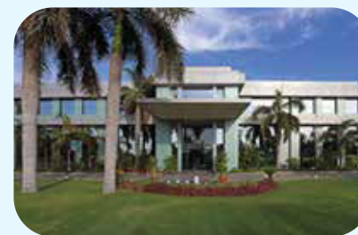
Harsha Engineers International Limited Changodar Plant
