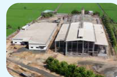
Harsha Engineers Advantek Limited Bhayla Plant 1
