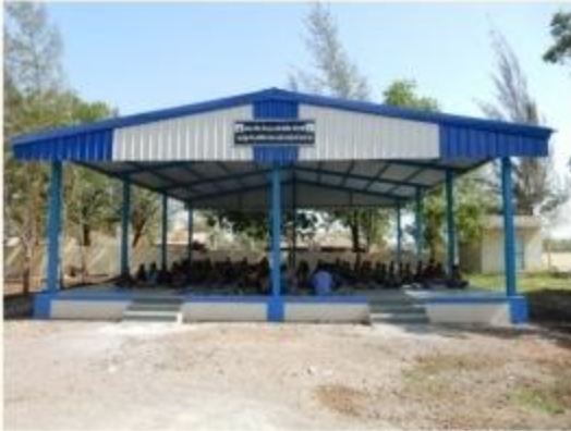
Multi purpose shed for Primary School of Nani Pardi, Ta.: Mangrol, Dist.: Surat.
