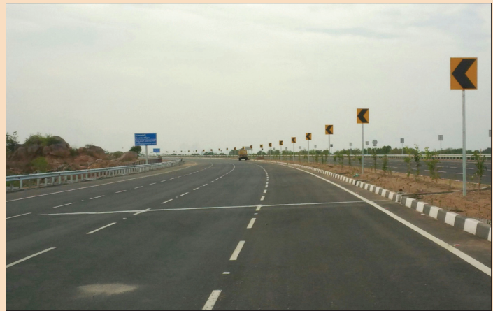
Hyderabad Outer Ring Road Project, Telangana
