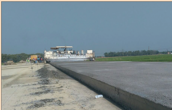
Cement Lining work in progress at Varanasi
