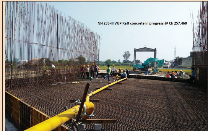
Raft concrete in progress at Varanasi
