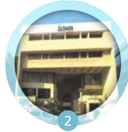
Fortis Hospital, C.G. Road, Bengaluru
