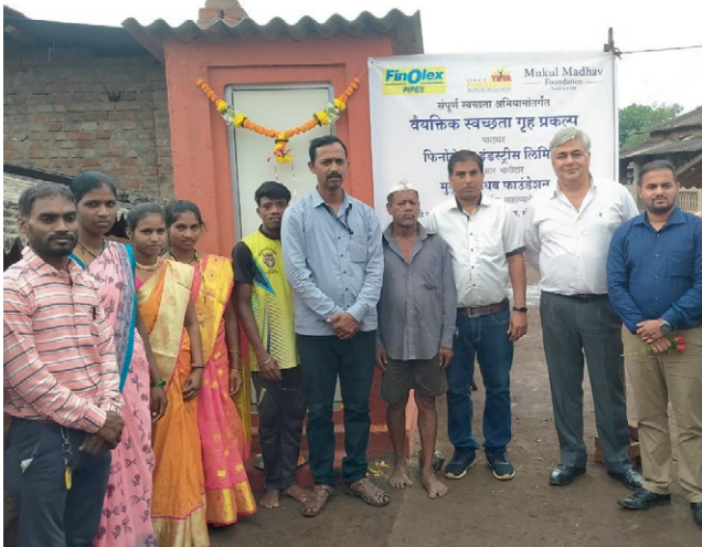
► Toilet construction at Palghar, Maharashtra
