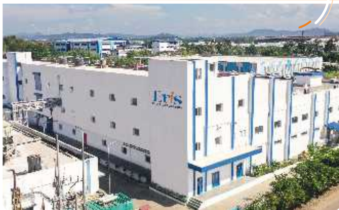
Guwahati Manufacturing Facility
