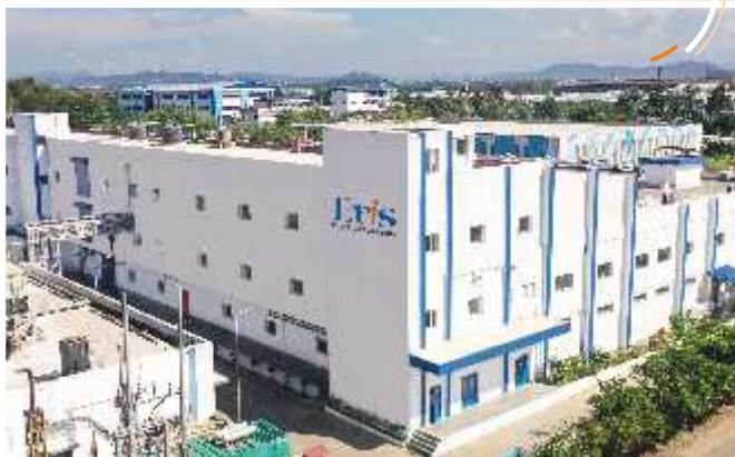
Guwahati Manufacturing Facility
