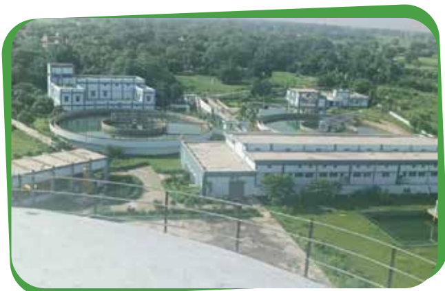
80 MLD Water Treatment Plant Unnao (Uttar Pradesh)
