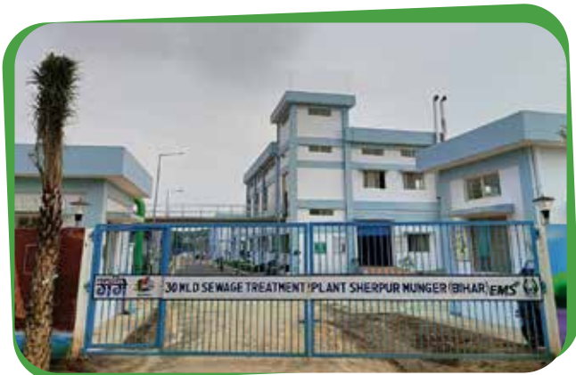
30 MLD Sewage Treatment Plant, Munger (Bihar)
