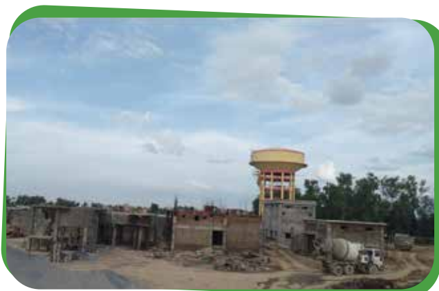
Hanumangarh Sewerage Work (Rajasthan)
