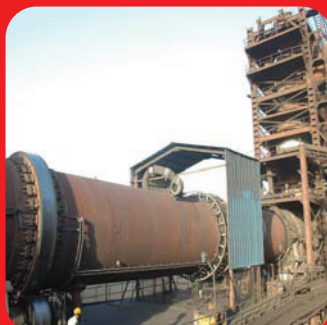
Coal Based DRI Plant
