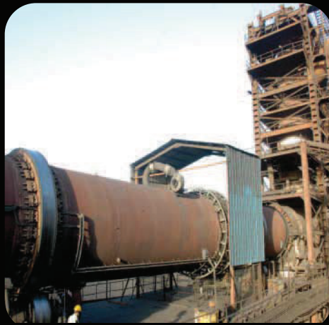
Coal Based DRI Plant
