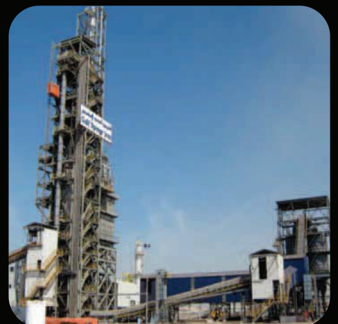
Gas based DRI Plant
