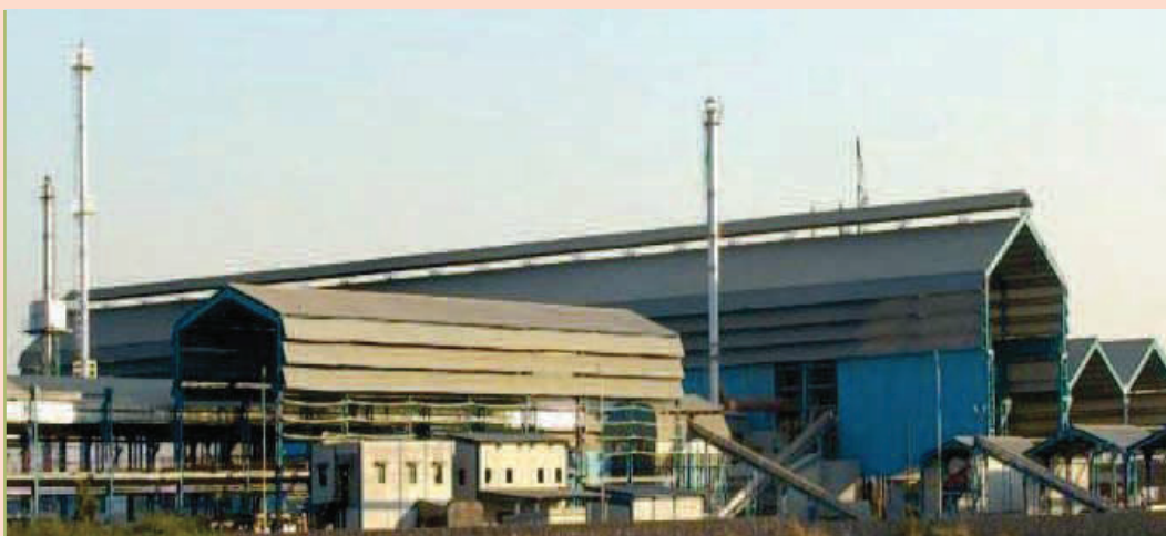
Plant at Samakhiyali, Kutch
