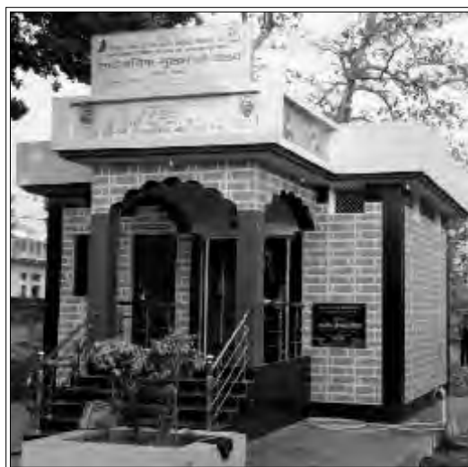
Community toilet in Ghazipur, Uttar Pradesh
