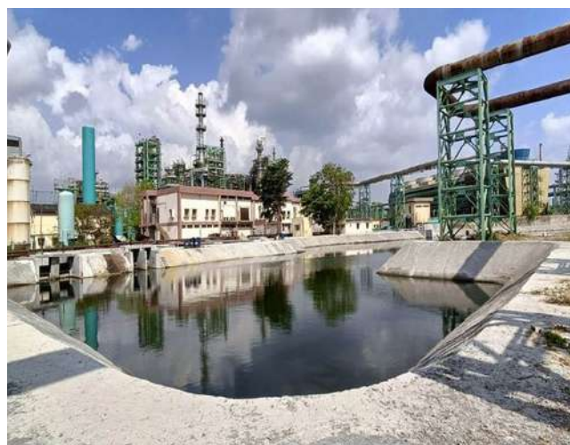
New Storm Water pond at Ref-I/II area
