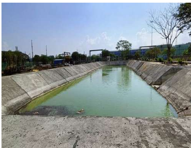
New Storm Water pond at Ref-III area
