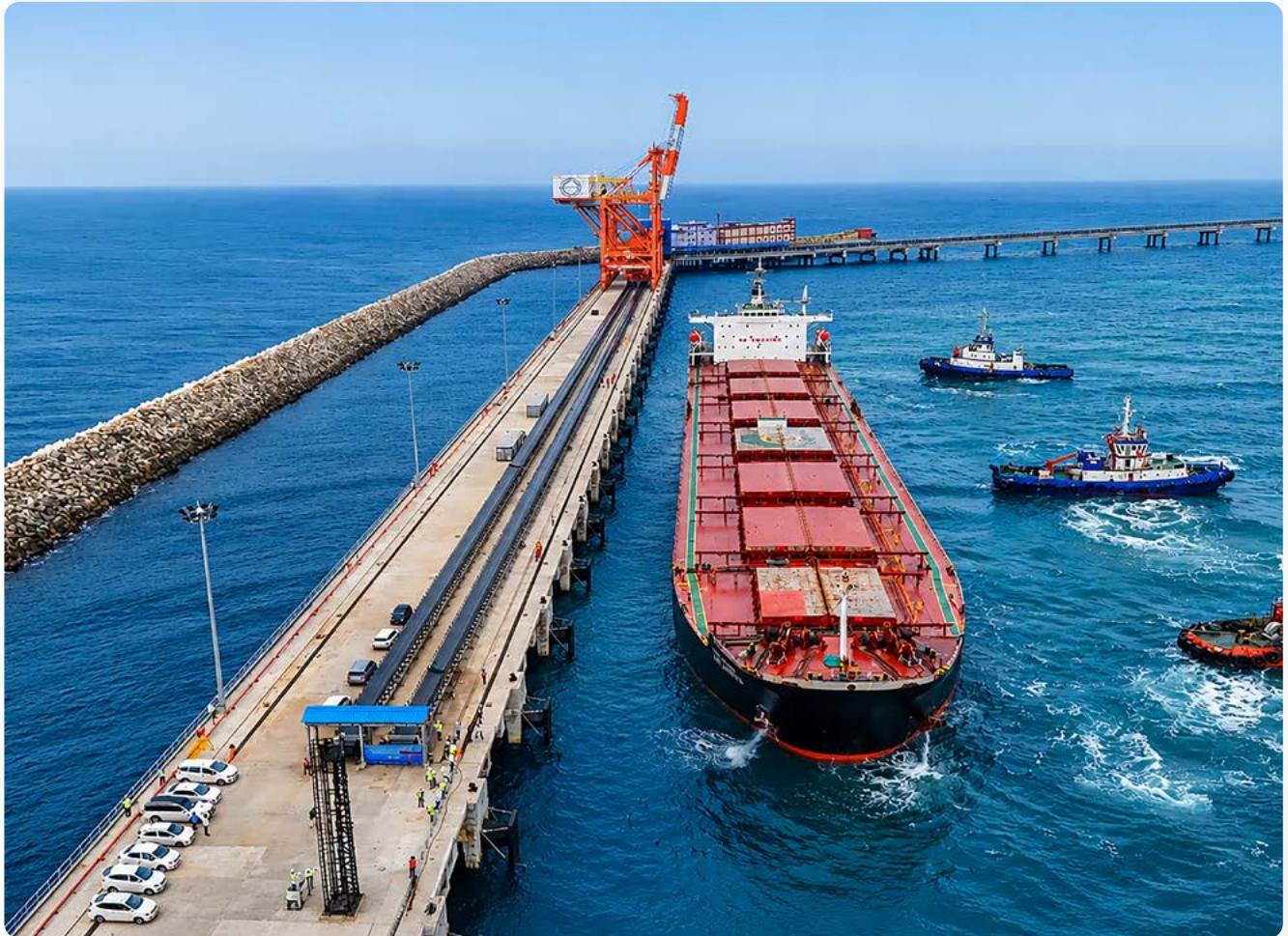
▲ Udangudi Marine Project in Tamil Nadu
