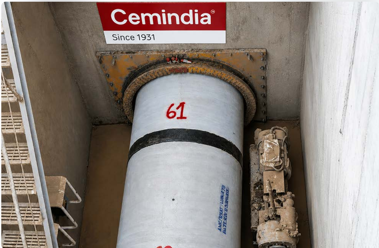
▲ Ahmedabad Micro-tunnelling Project in Gujarat
