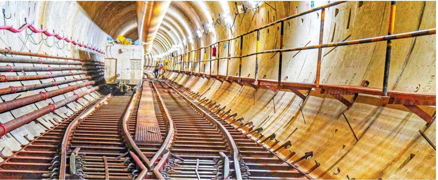
▲ Chennai Underground Metro Tunnel in Tamil Nadu
