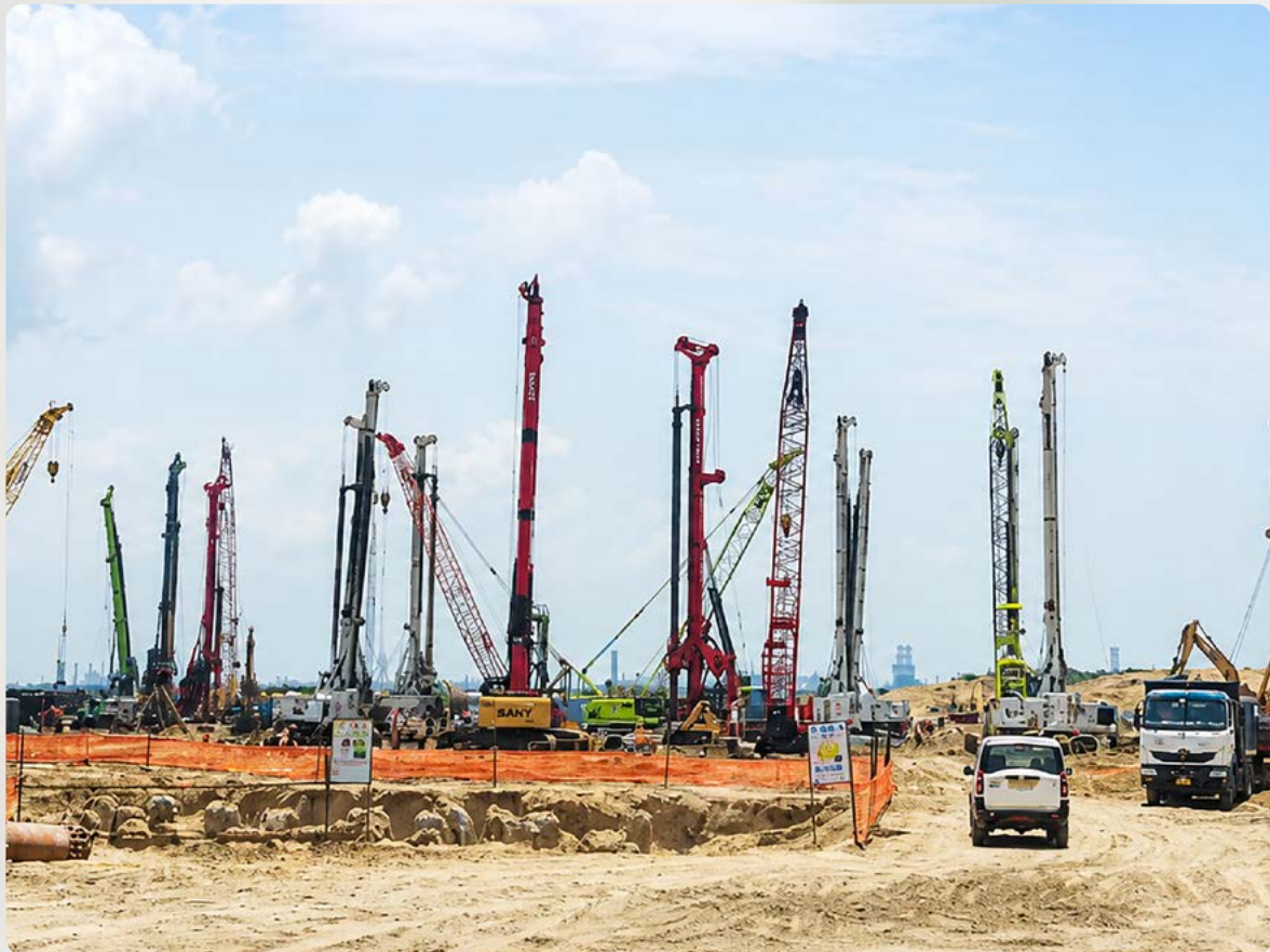
▲ Piling Work at JSW Utkal in Odisha
