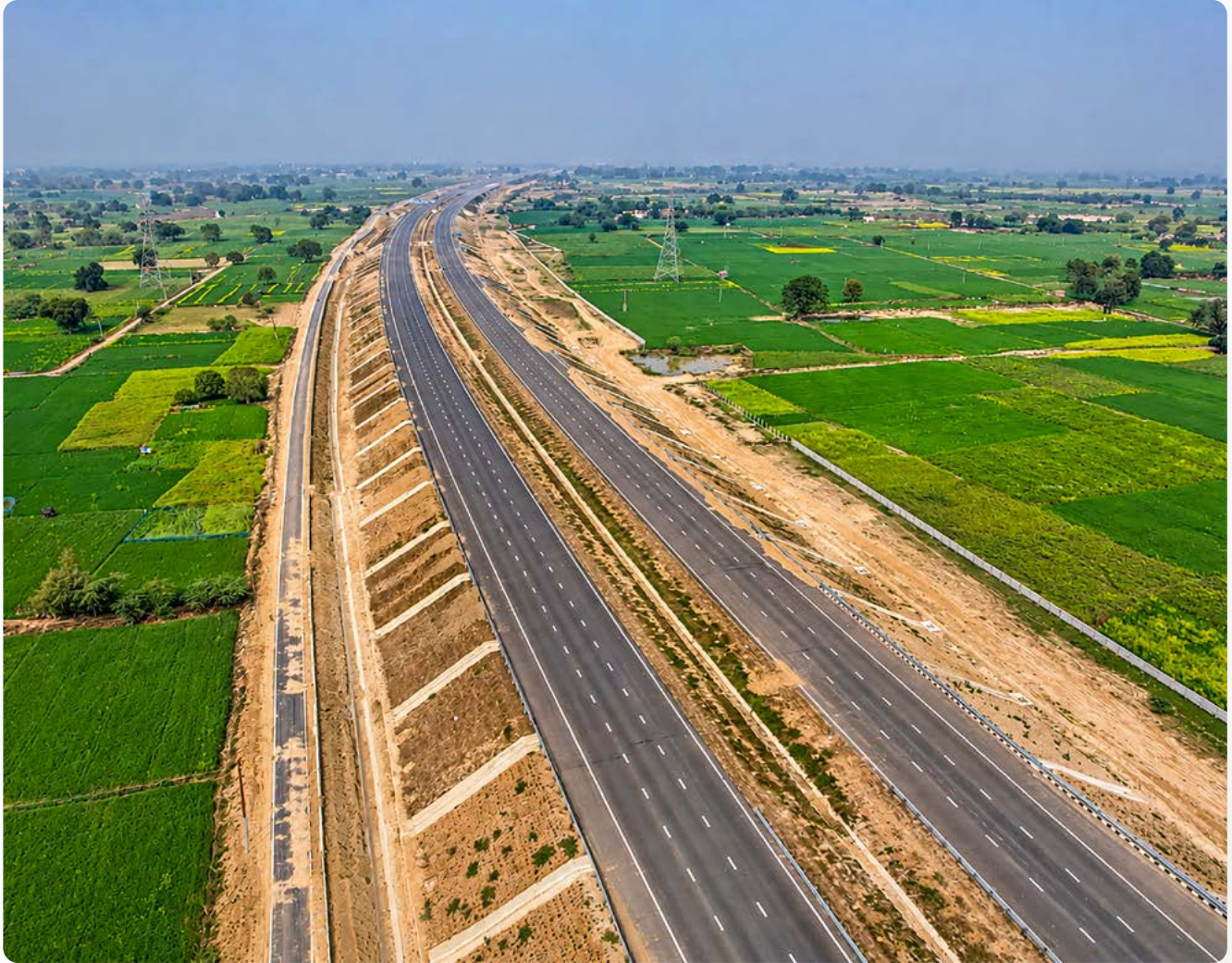
▲ Ganga Expressway Road Project in Uttar Pradesh
