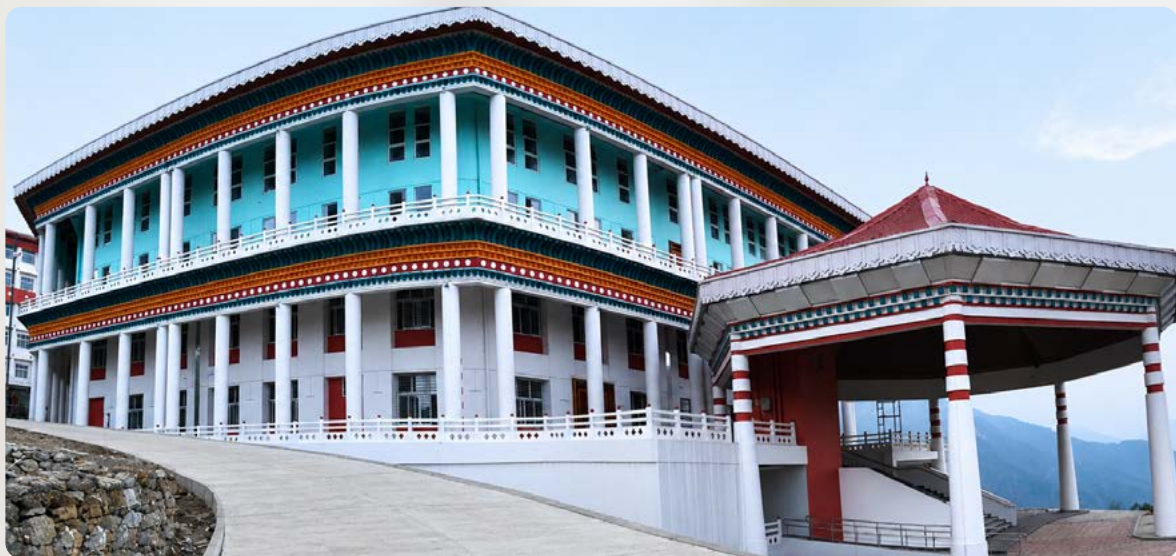
▲ University Building in Yangang, Sikkim
