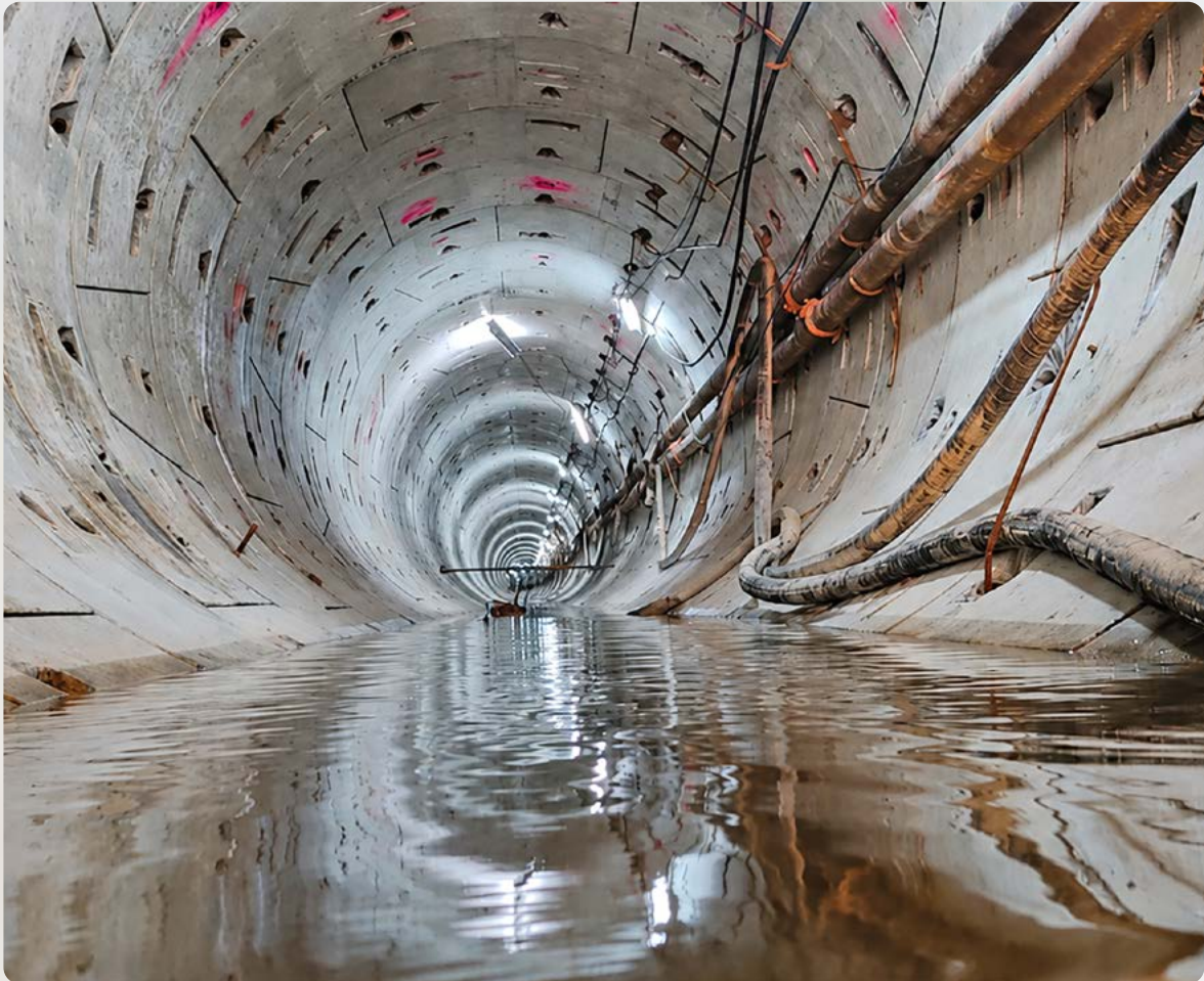
▲ MCGM Micro-tunnelling Project in Maharashtra
