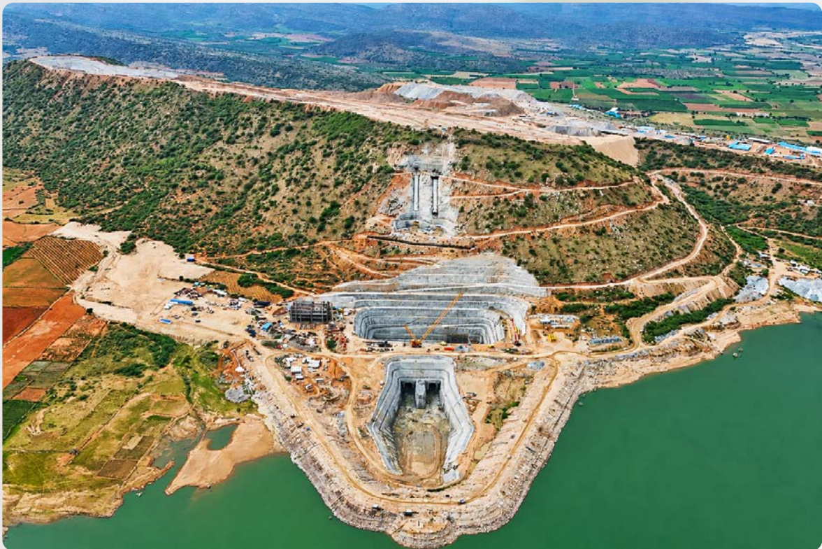
▲ Chitravathi Pumped Storage Project in Andhra Pradesh
